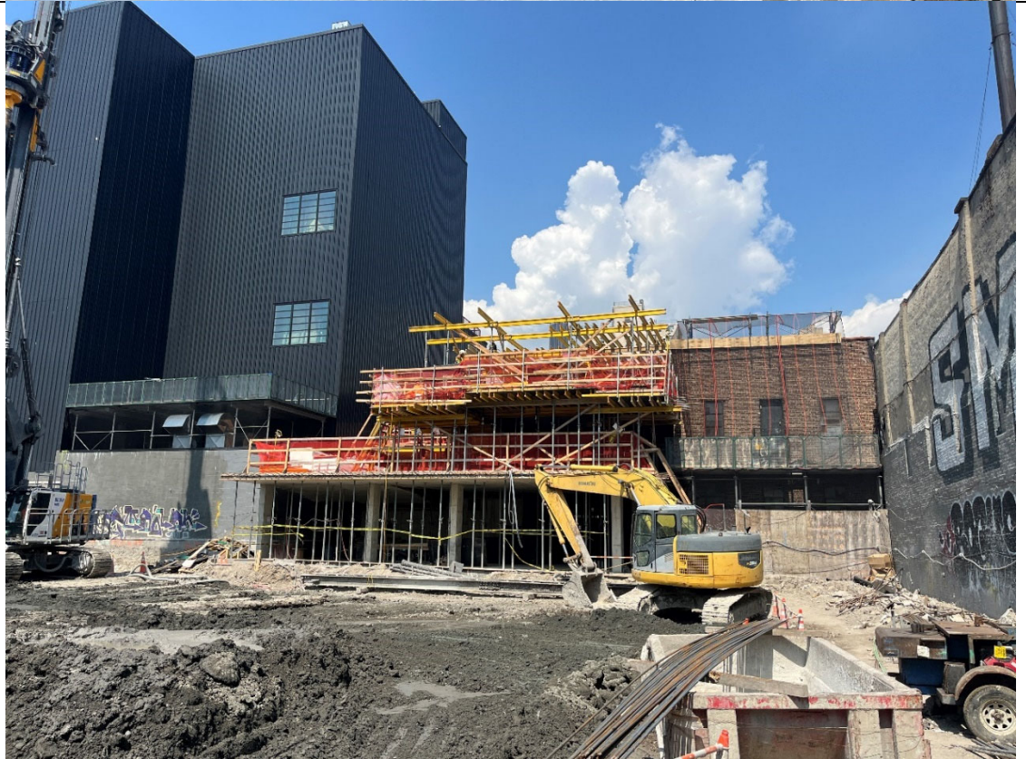
Photo 4- Representative photo of Concrete Courses in the Butler Corridor.
