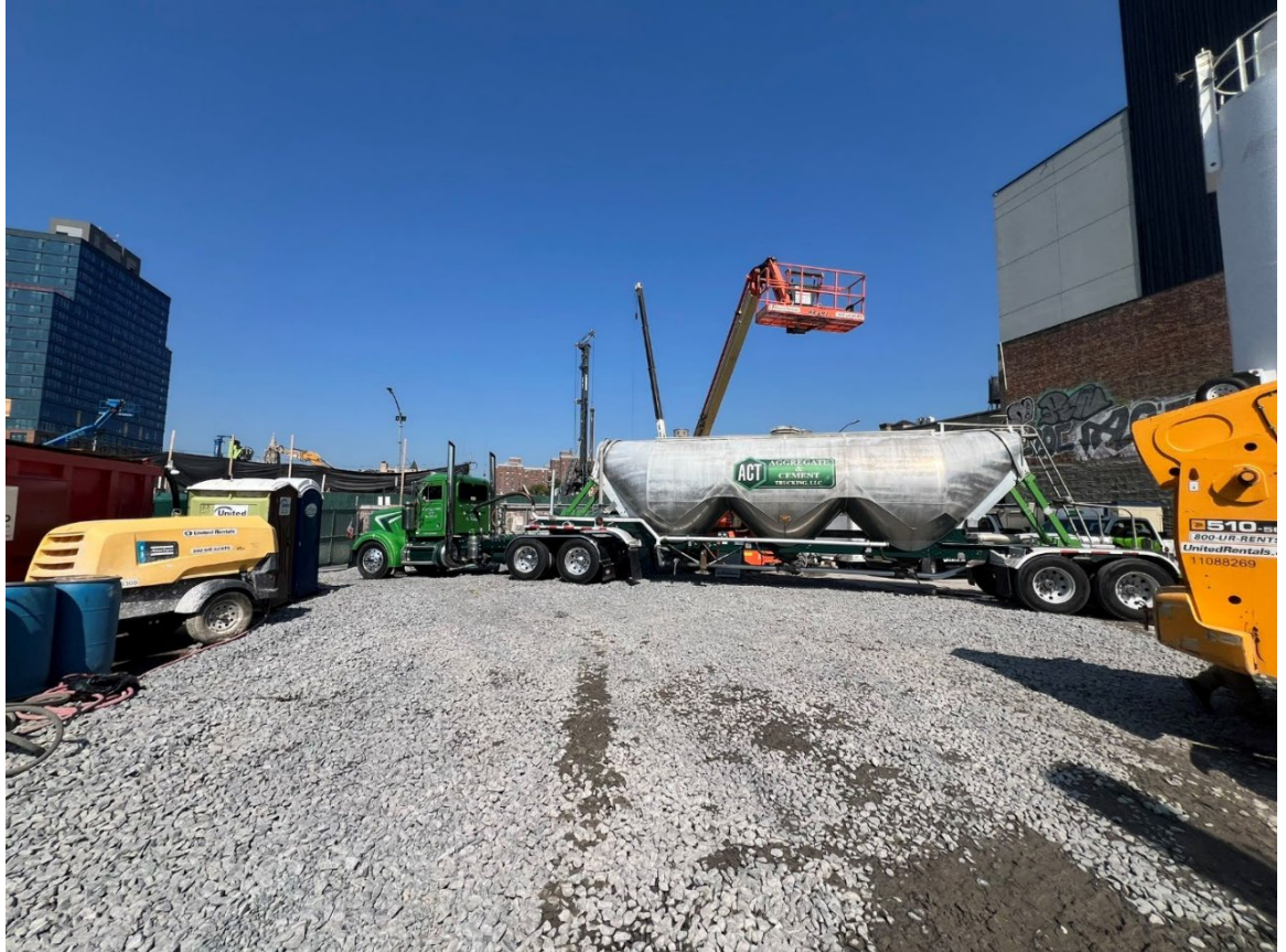
Photo 2- Representative photo of Cascade receiving a slag delivery.
