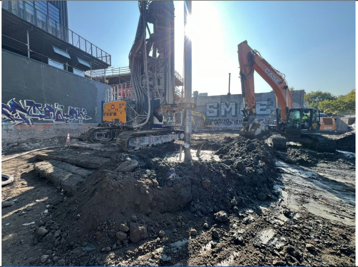
Photo 1- Representative photo of ISS pilot column over-drill with 6' auger.
