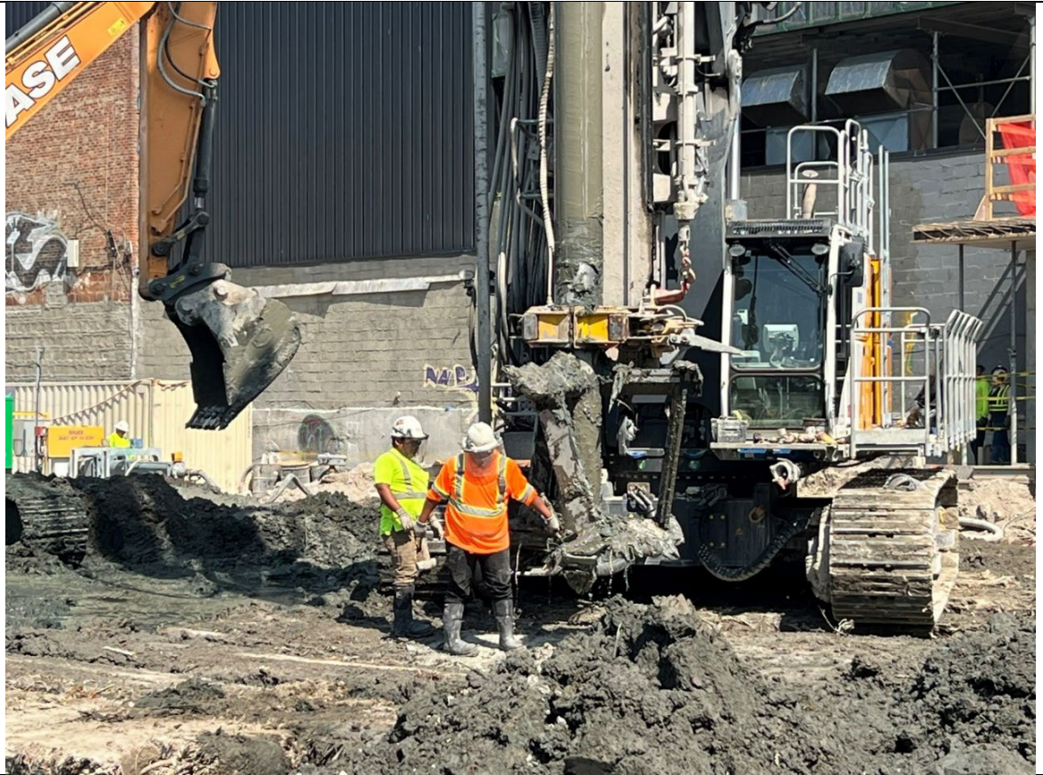
Photo 3- Representative photo of Cascade changing teeth on the auger.
