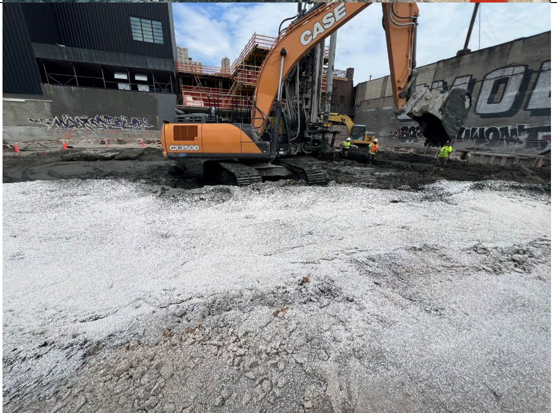
Photo 4- Representative photo ATMOS foam sprayed in the work area.
