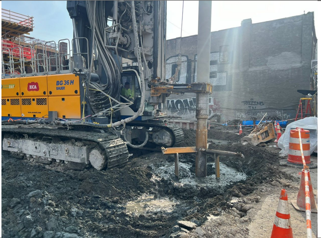
Photo 3- Representative photo of drilling an ISS column.
