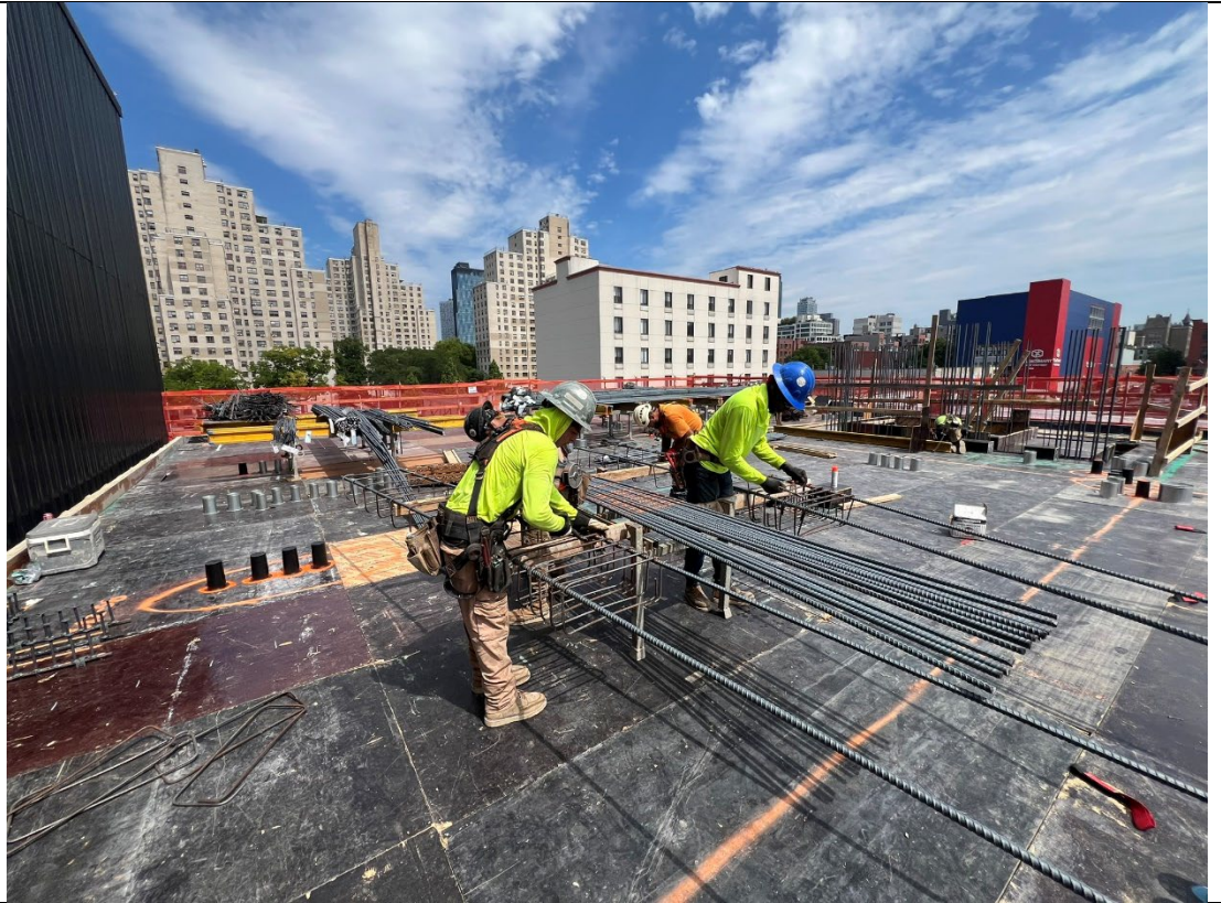
Photo 5- Representative photo of super structure work.
