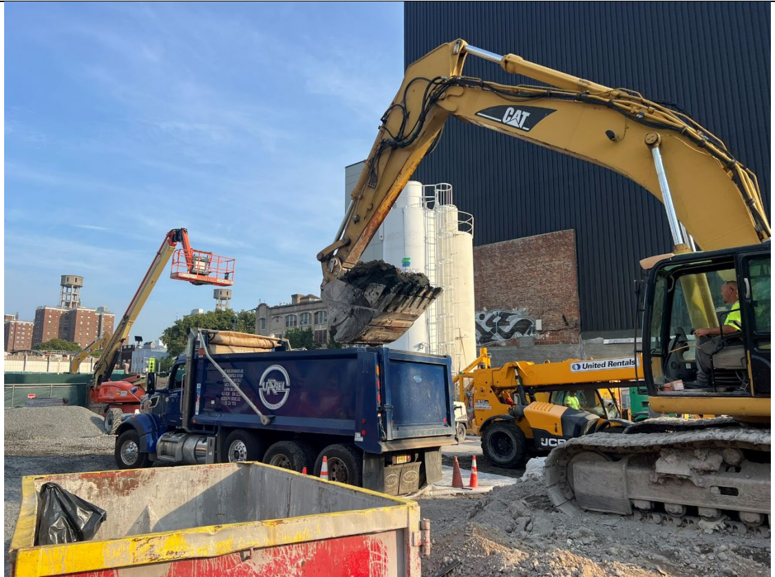
Photo 1- Representative photo of truck being loaded with swell material for offsite disposal.
