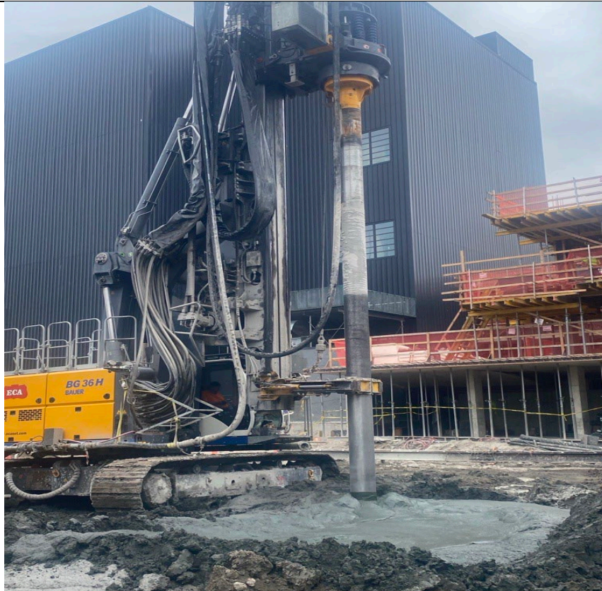
Photo 1- Representative photo of ISS column installation.
