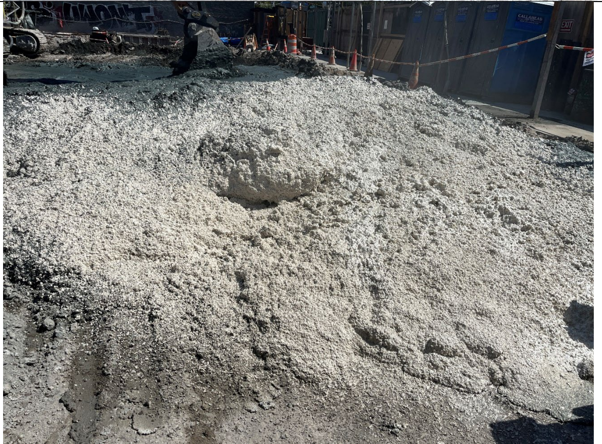
Photo 2- Representative photo of ATMOS foam applied to ISS work area.
