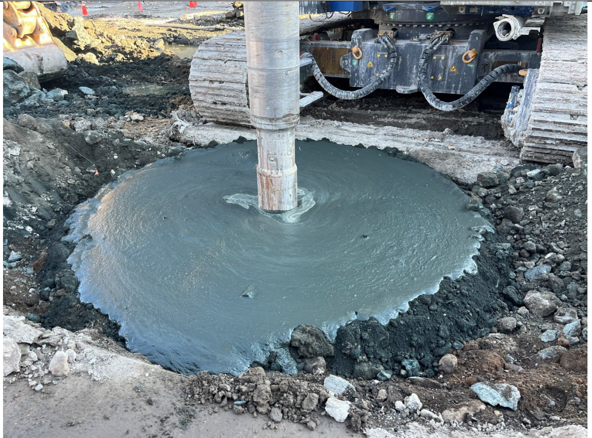
Photo 1- Representative photo of ISS column installation.
