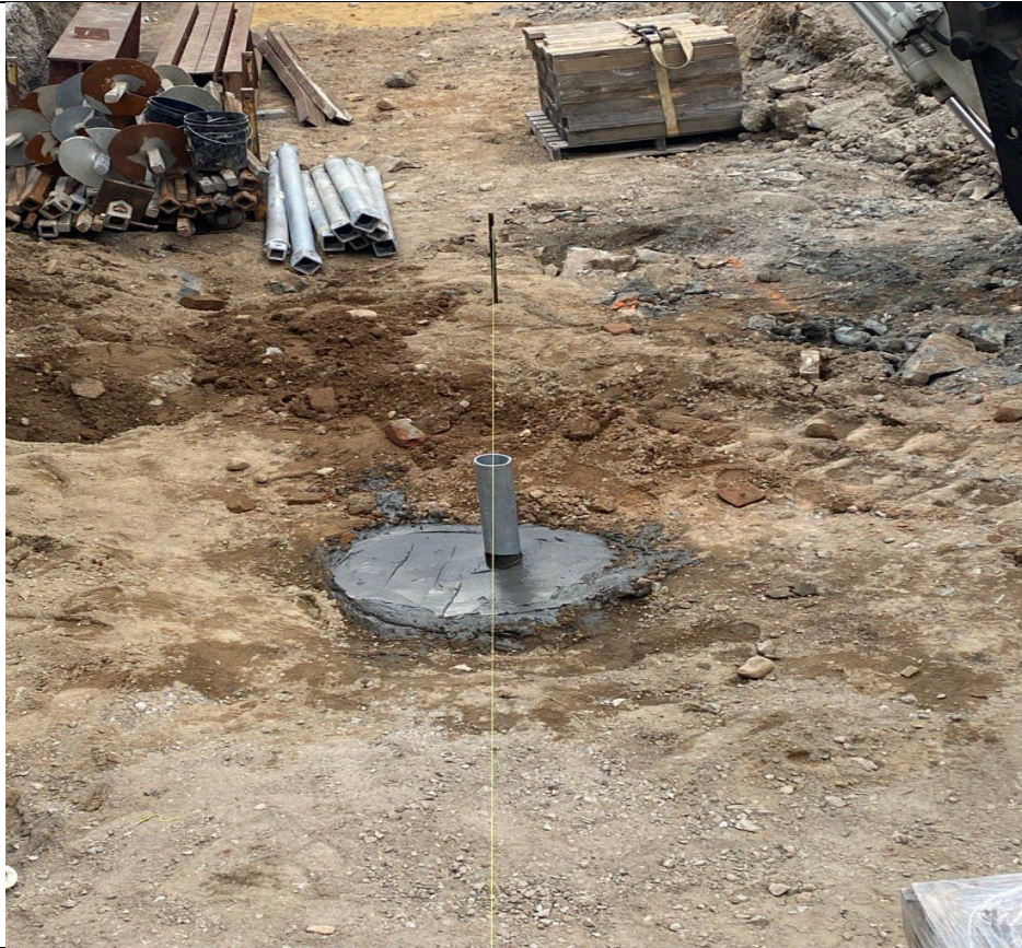
Photo 3- Representative photo of test- piles installed in the Con Ed vault.
