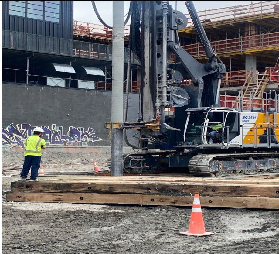
Photo 1- Representative photo of ISS column installation.
