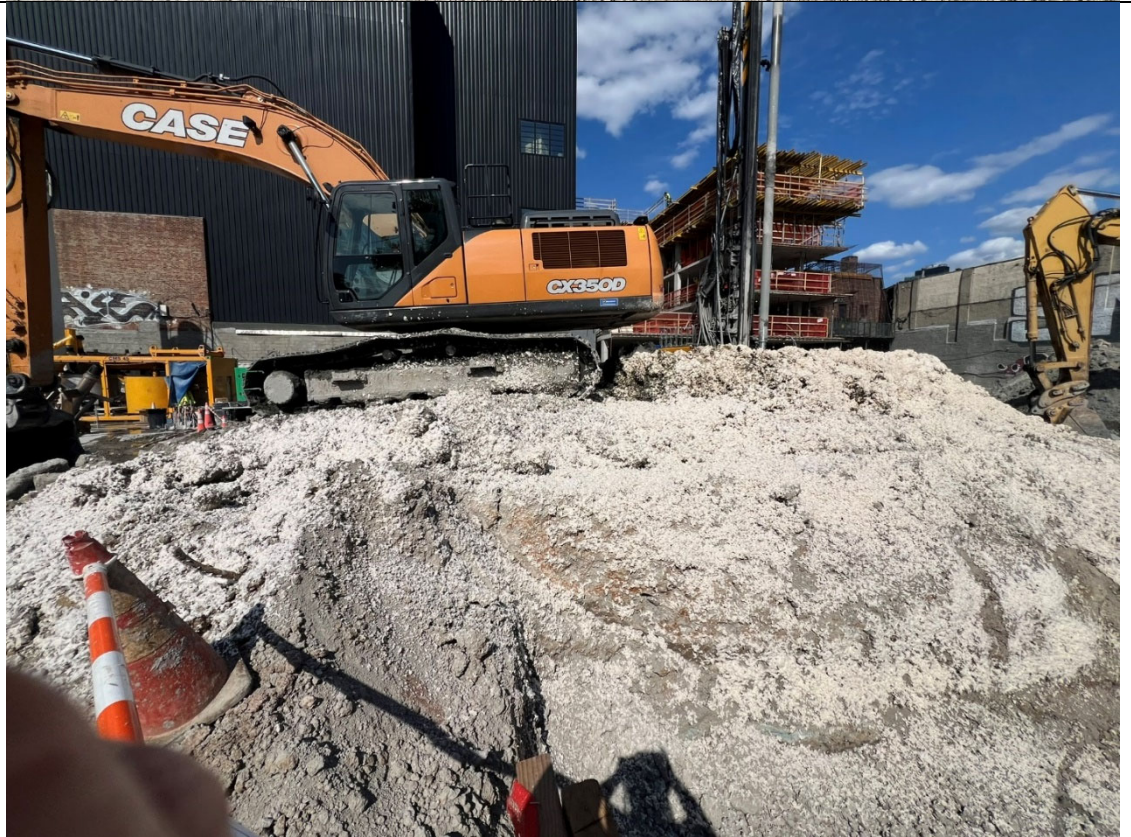
Photo 4- Representative photo of stockpile sprayed with foam at the end of the day.
