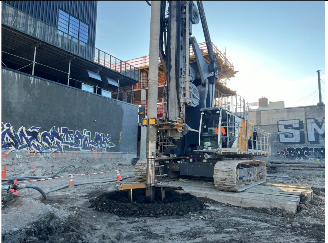
Photo 1- Representative photo of ISS column installation.
