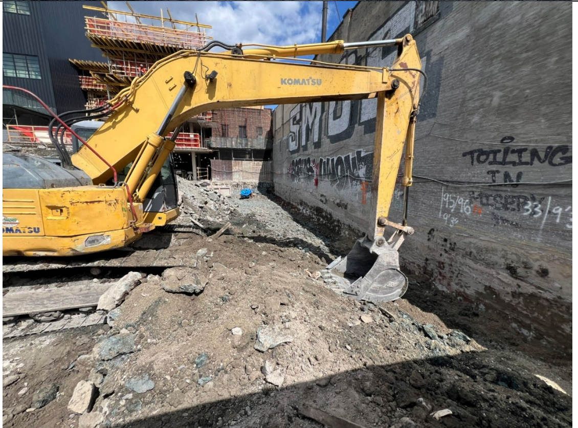
Photo 2- Representative photo of excavation for bottom of slab.
