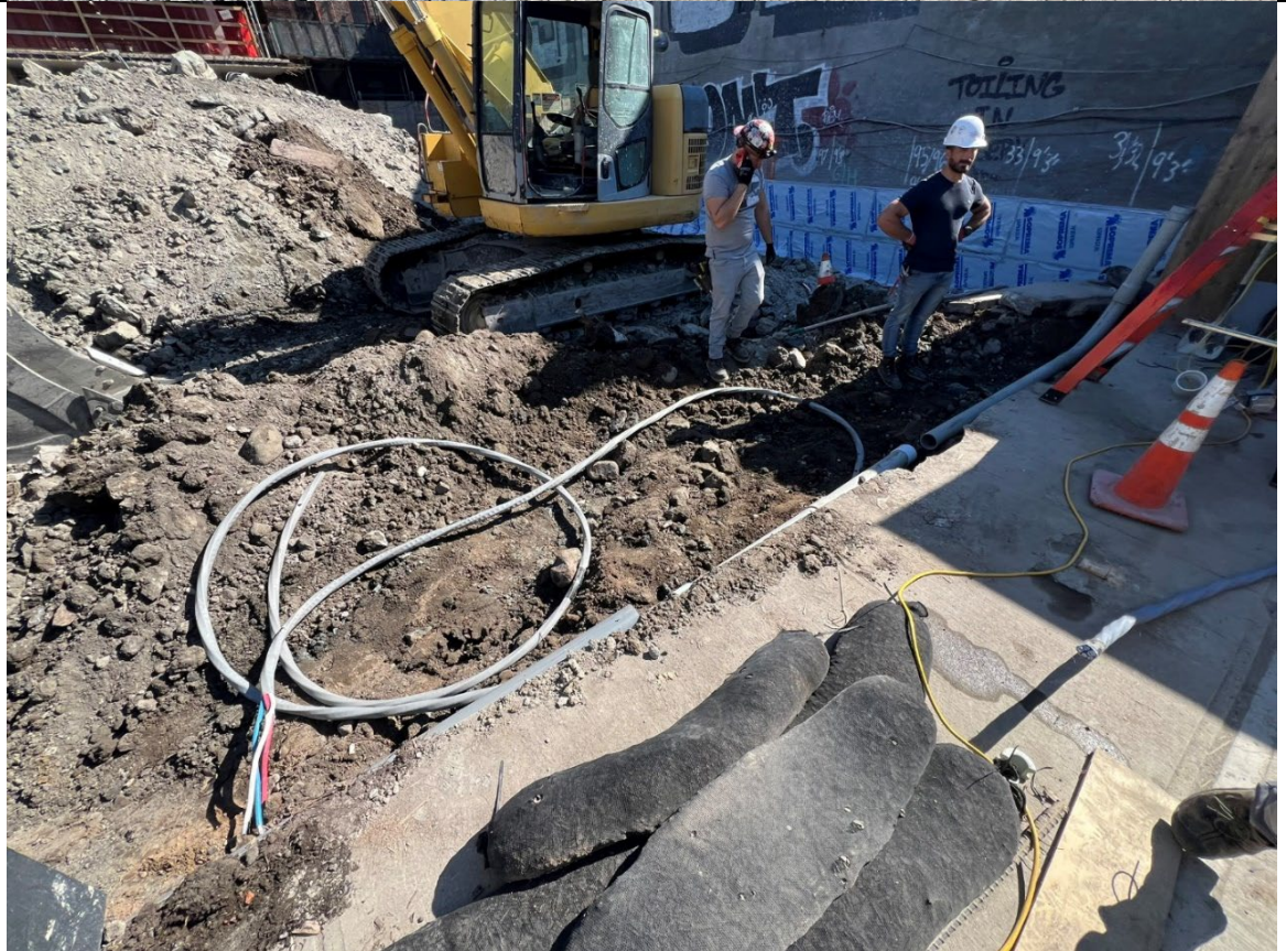
Photo 4- Representative photo of electricians installing underground utilities.
