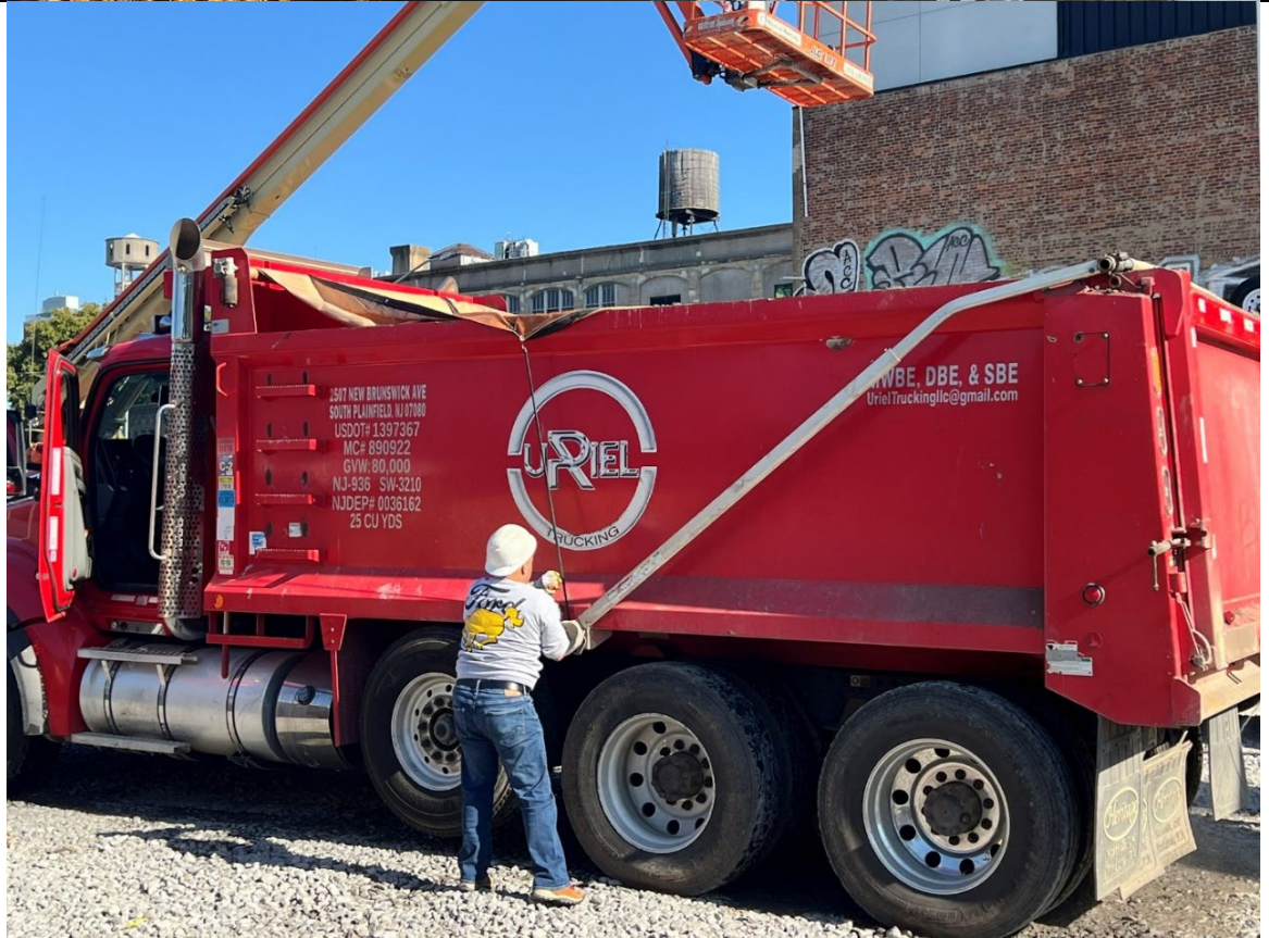
Photo 2- Representative photo of straps being secured on the side of a truck prior to exiting the Site.
