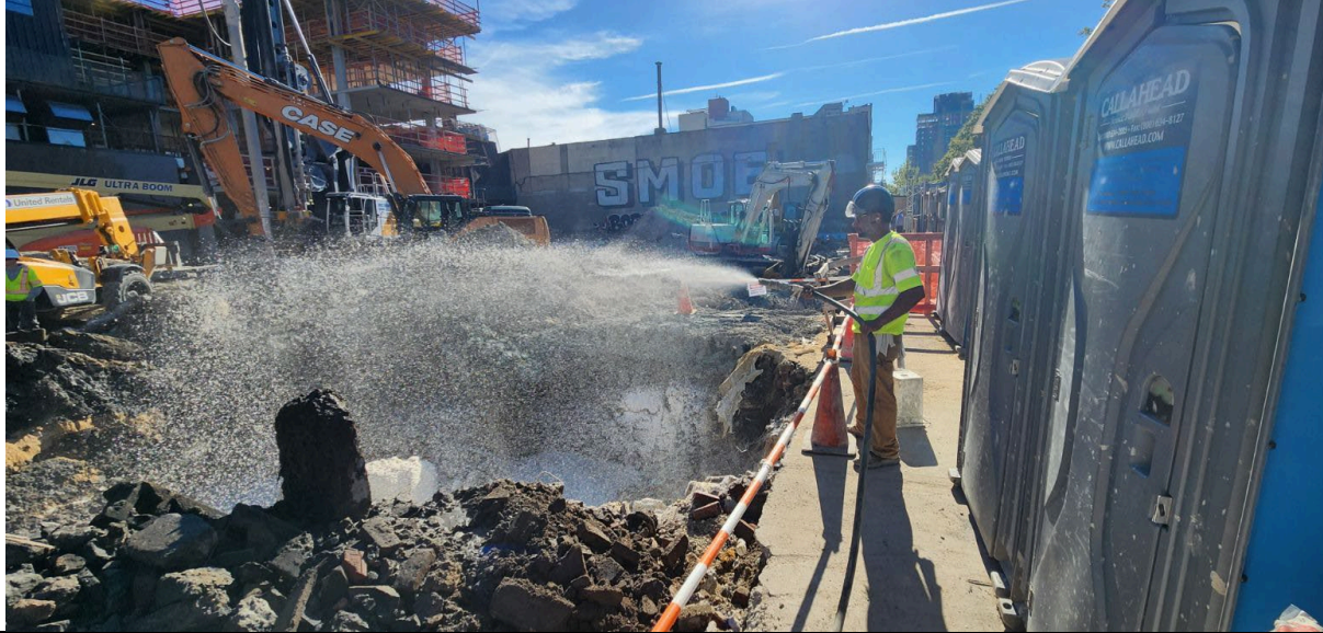
Photo 6- Representative photo of ATMOS foam being sprayed in the tank area.
