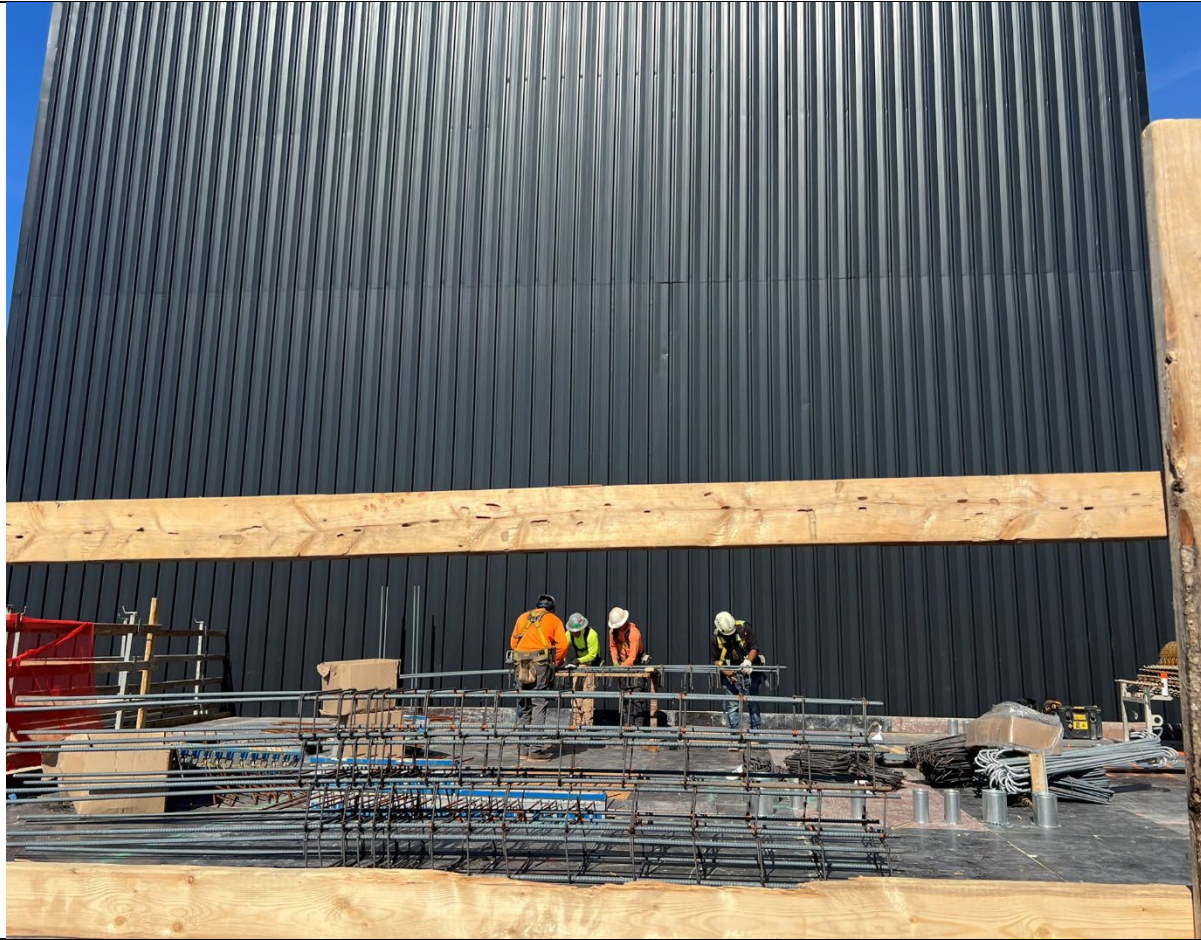
Photo 7- Representative photo of super structure work.
