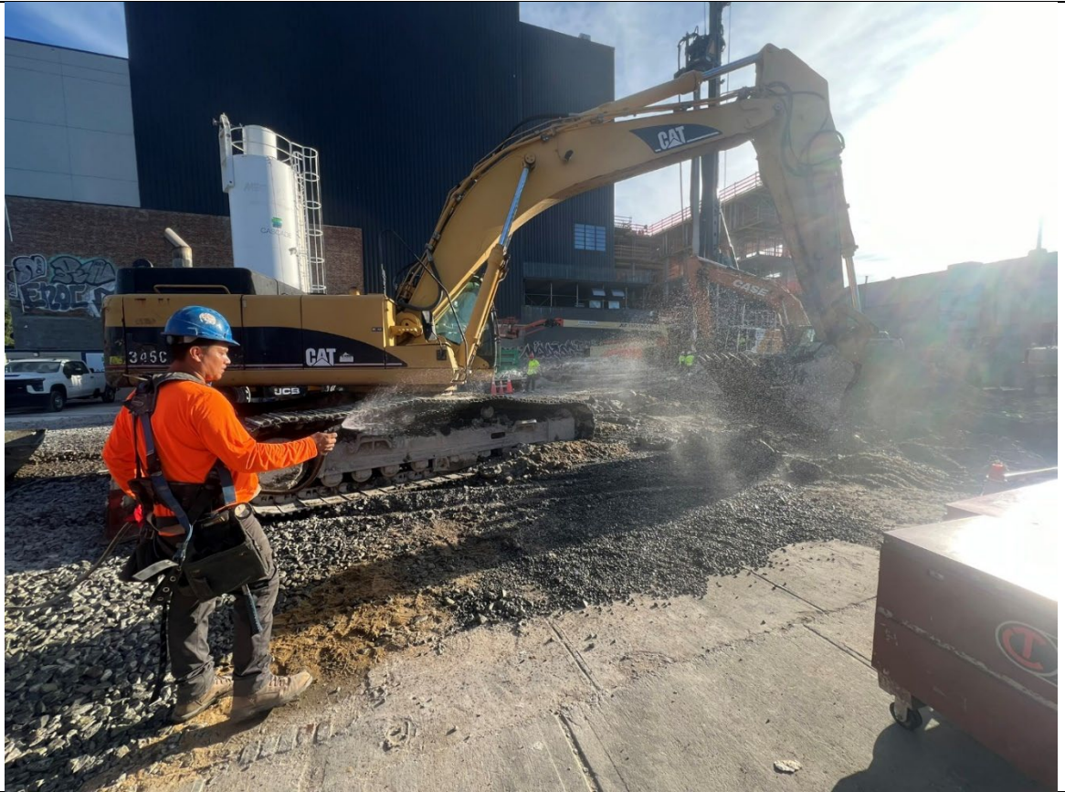
Photo 3- Representative photo of dust suppression being used while excavating.
