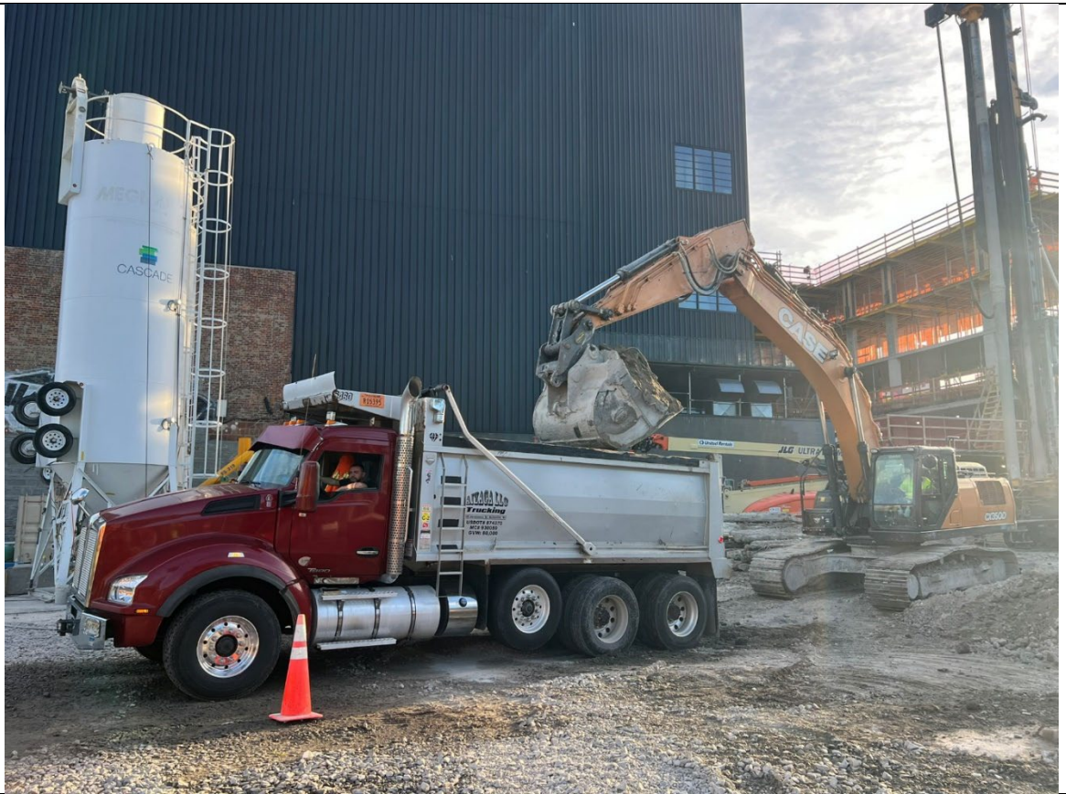
Photo 1- Representative photo of swell material being loaded out for removal offsite.
