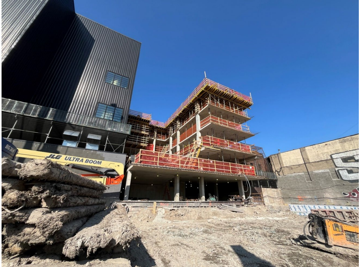
Photo 6- Representative photo of Butler Corridor superstructure.
