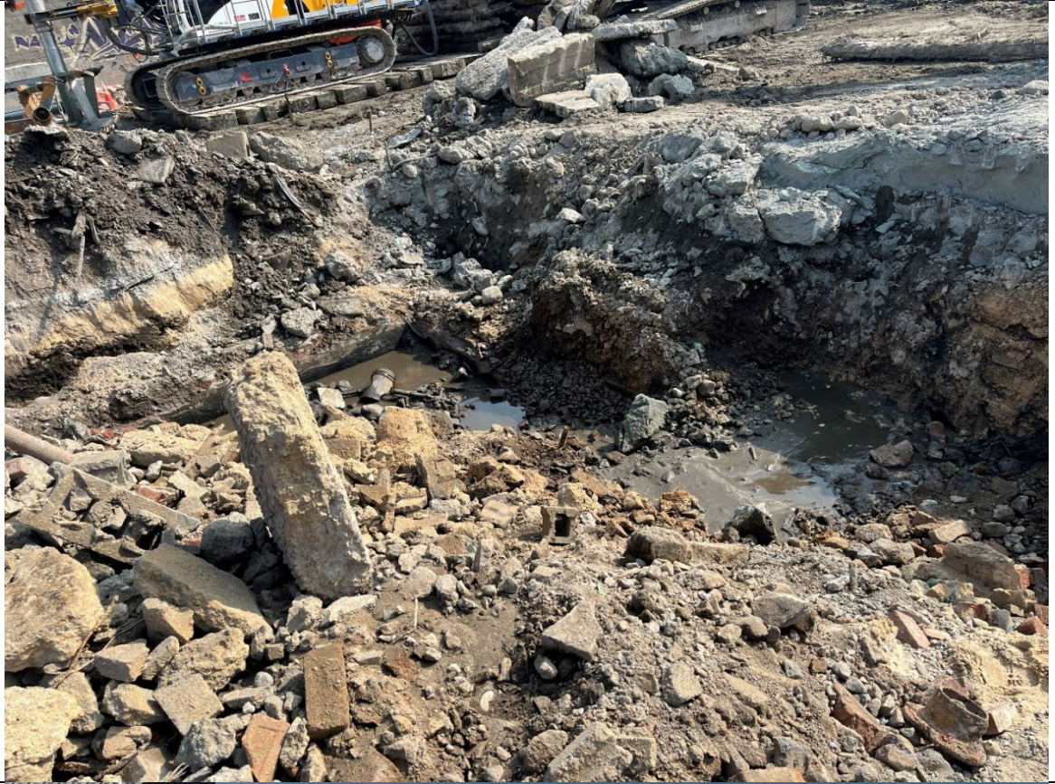
Photo 5- Representative photo of Tank 3 and Tank 4 graves.
