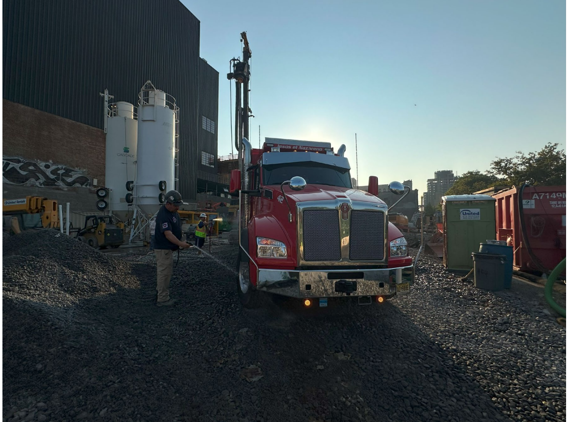
Photo 2- Representative photo of truck tires being washed before exiting site.
