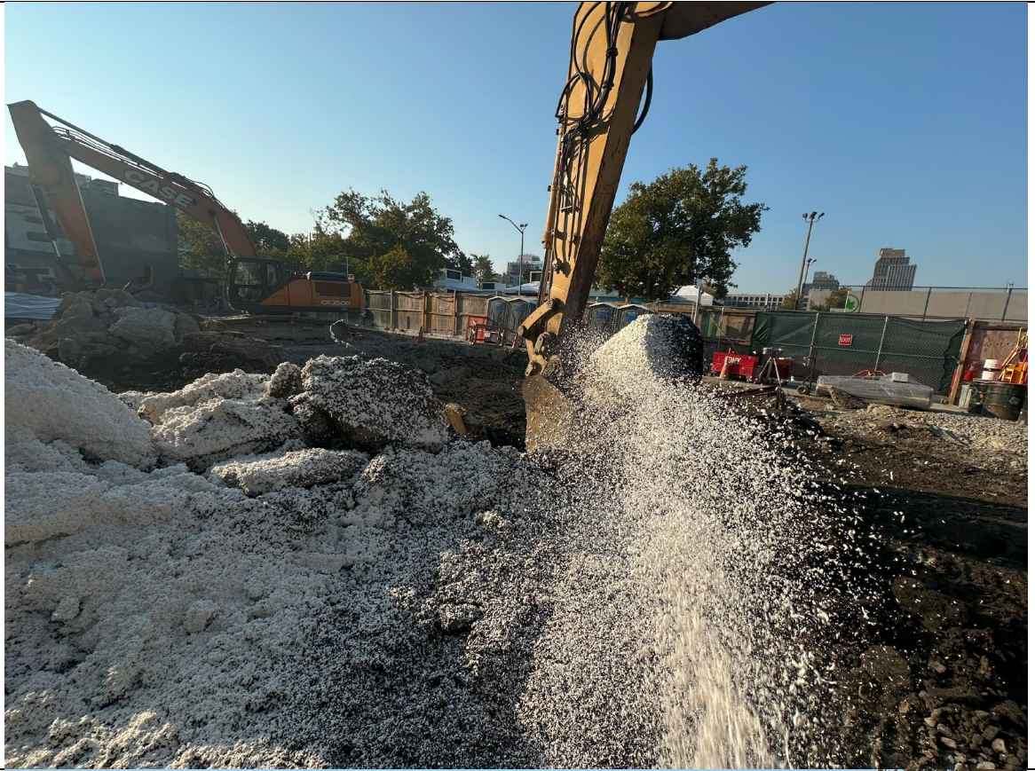
Photo 3- Representative photo of Atmos foam being used while excavating.
