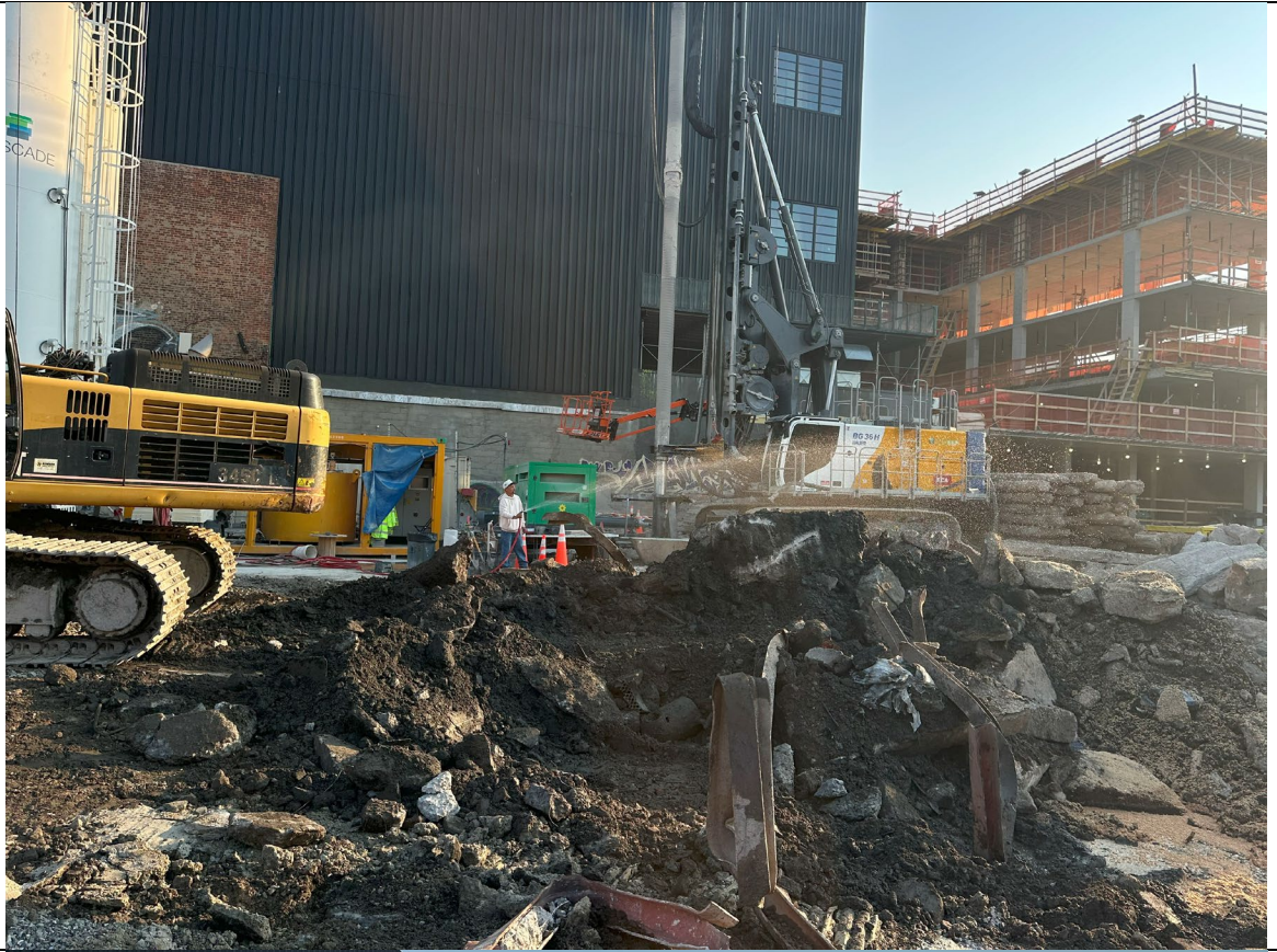
Photo 1- Representative photo of water being used for dust suppression.
