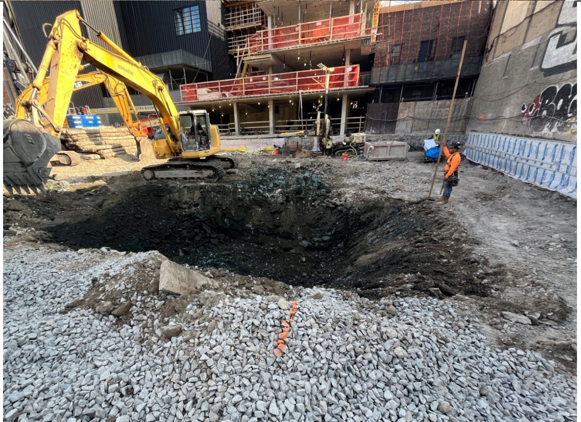
Photo 2- Representative photo of Concrete Courses excavating elevator pit.
