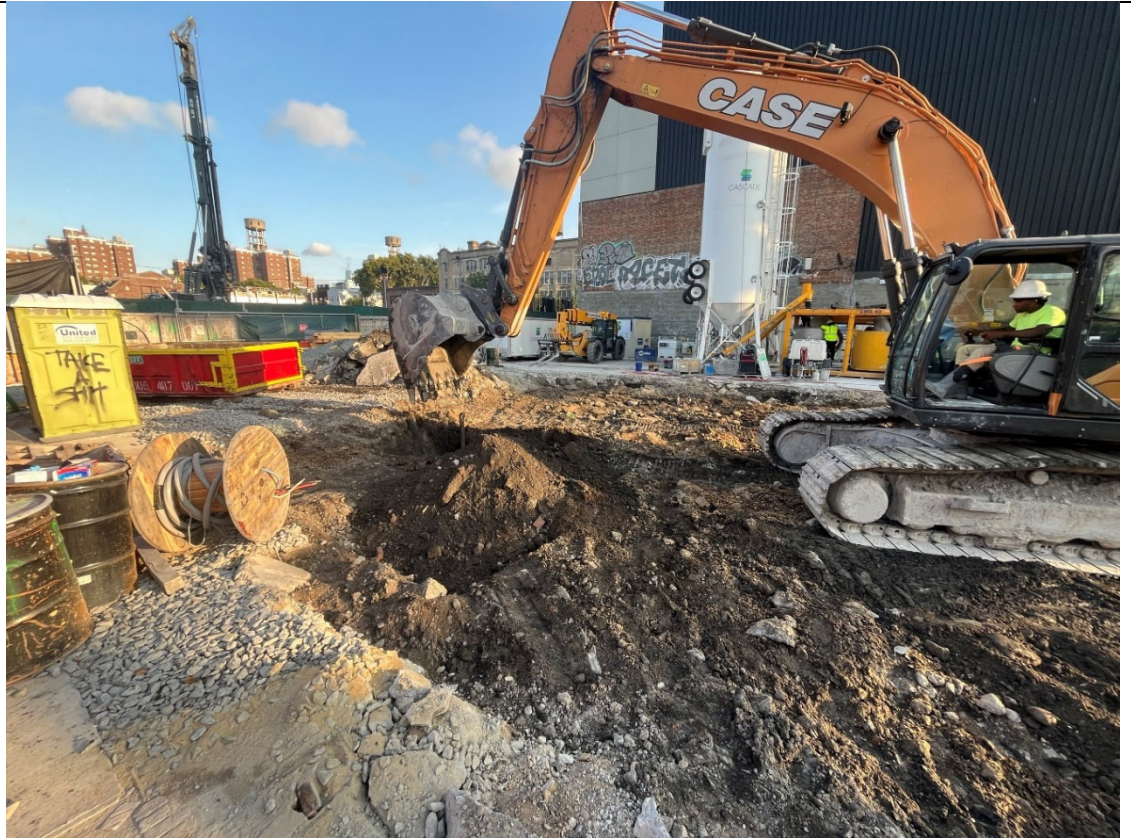
Photo 1- Representative photo of Cascade completing 4' cut for endpoint sampling.
