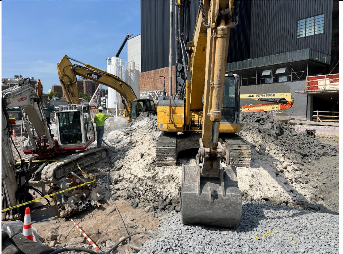
Photo 6- Representative photo of ATMOS foam application to ISS material stockpile.
