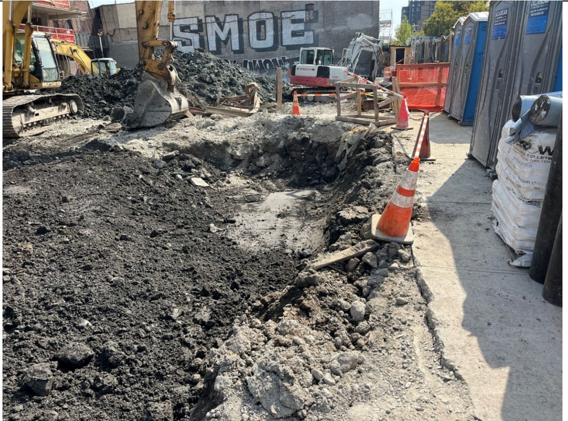
Photo 5- Representative photo of 4' cut in western portion of the site.
