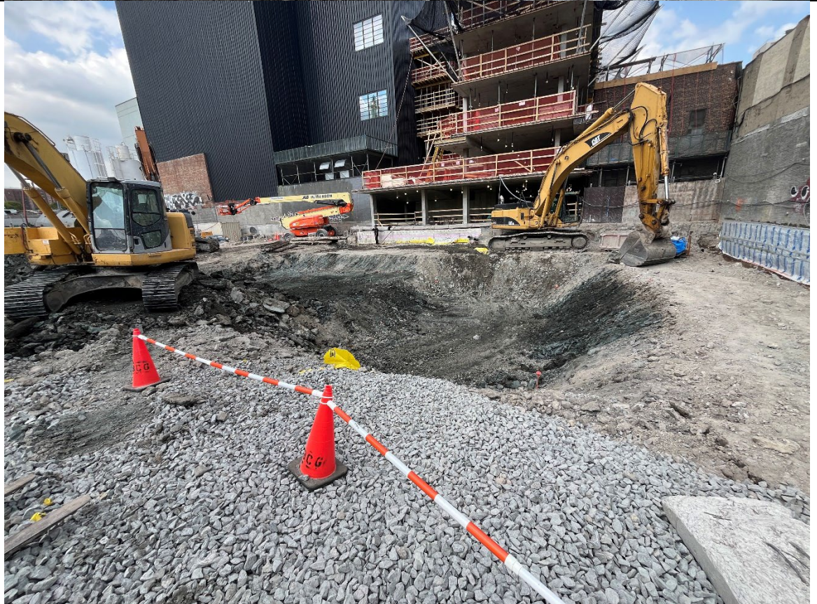
Photo 6- Representative photo of elevator pit in eastern portion of the site.
