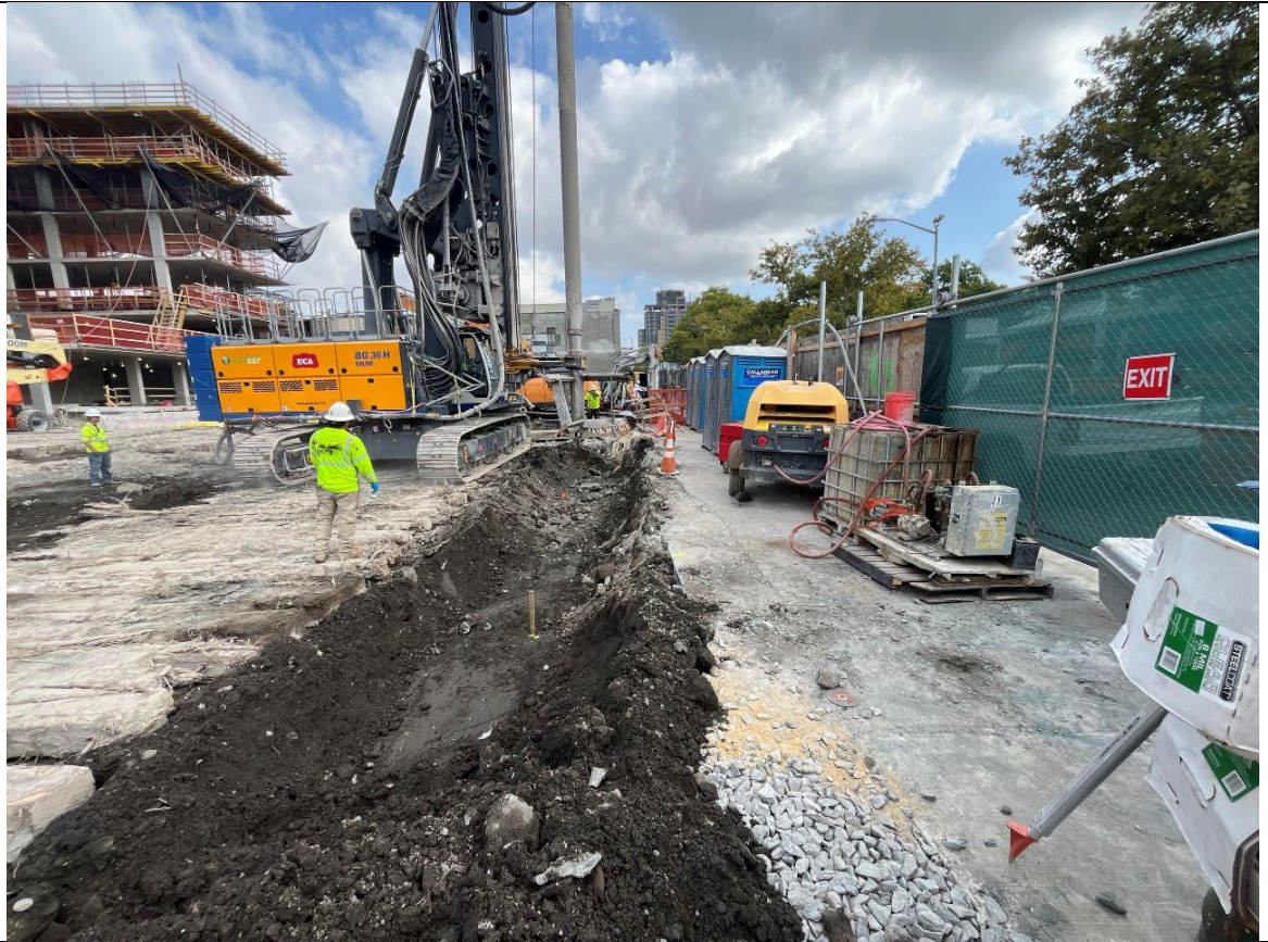
Photo 5- Representative photo of ISS columns marked out.
