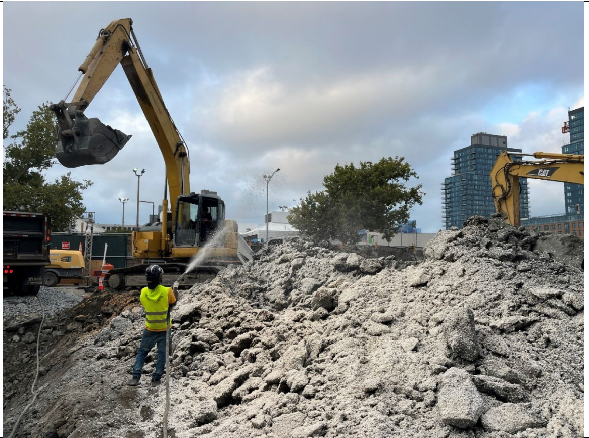
Photo 1- Representative photo of ATMOS Foam application during loadout.
