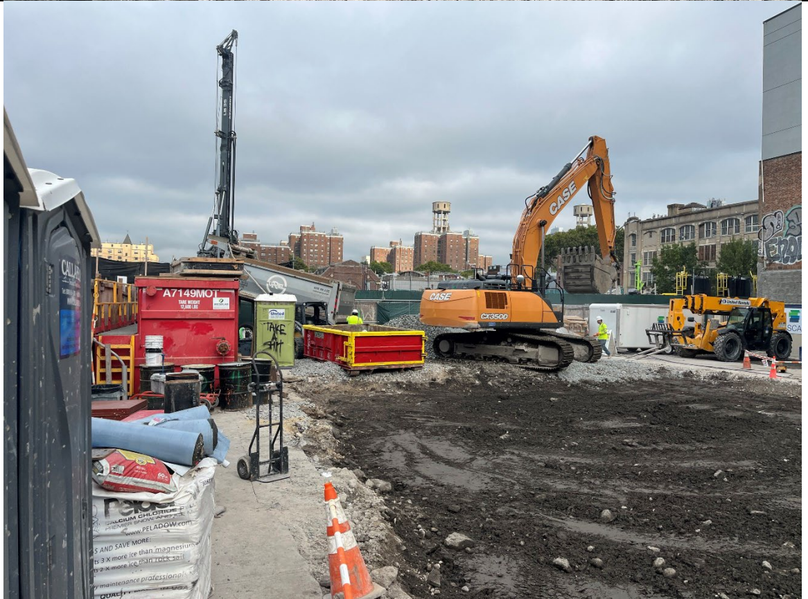
Photo 2- Representative photo of approved stone delivery for western trucking pad.
