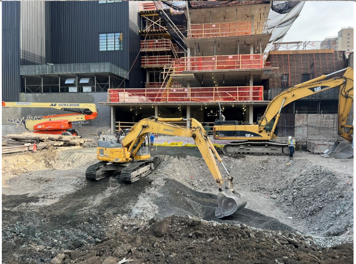
Photo 2- Representative photo of stone being laid down in the elevator pit.
