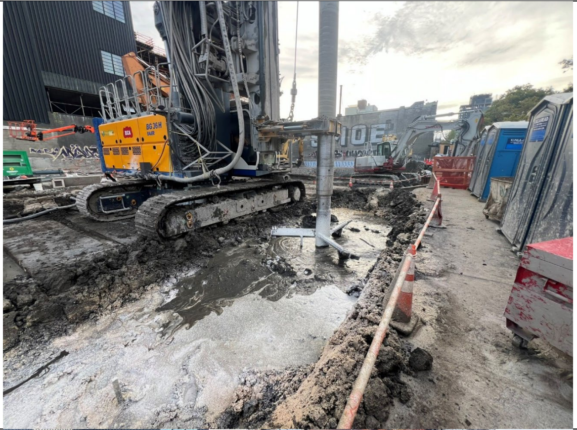
Photo 1- Representative photo of drilling ISS column.
