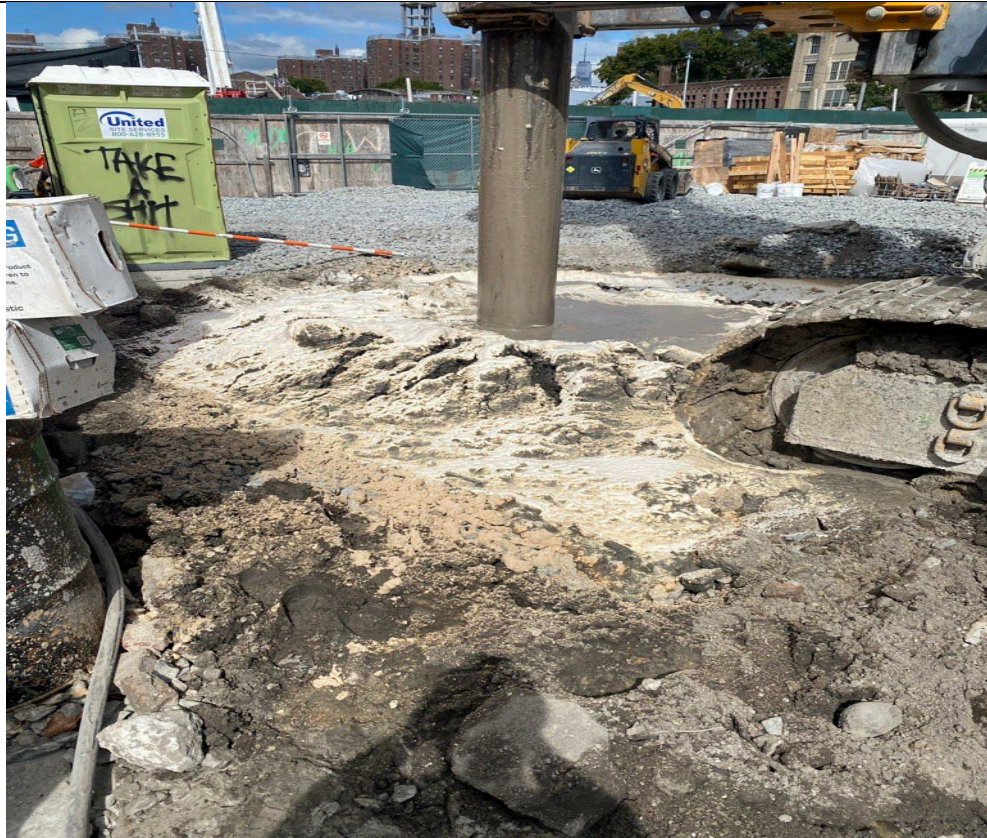
Photo 3- Representative photo of ATMOS foam applied to swell cuttings.
