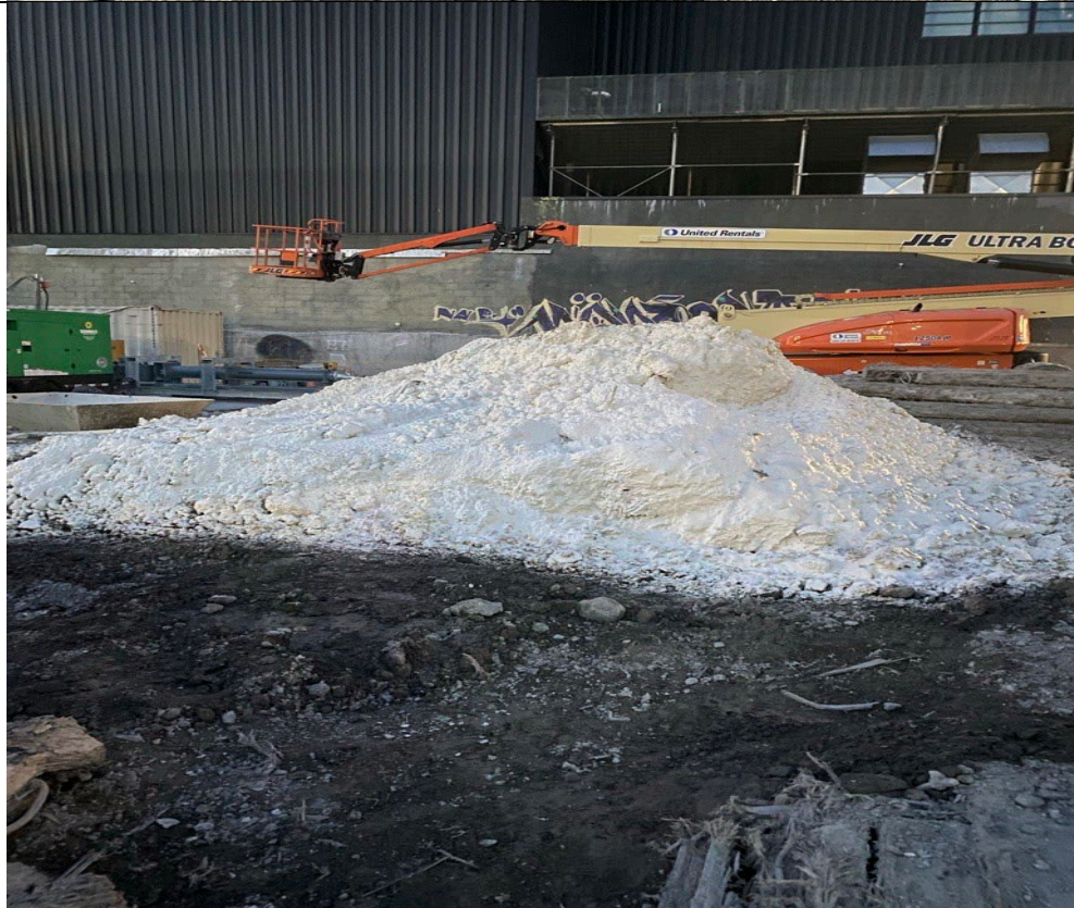
Photo 4- Representative photo of swell stockpile covered with ATMOS foam at the end of the day.
