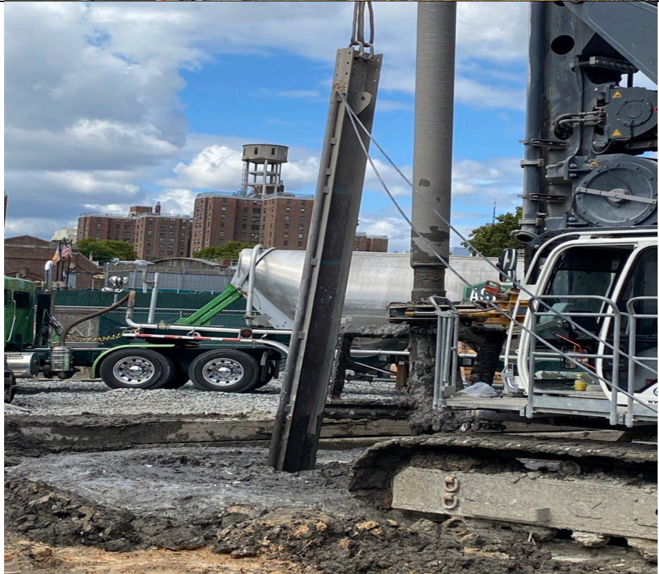
Photo 2- Representative photo of wet-mix sample collected from ~30' depth at Column 56.
