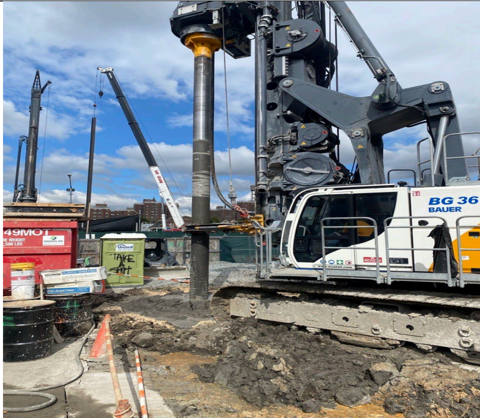
Photo 1- Representative photo of drilling ISS column.
