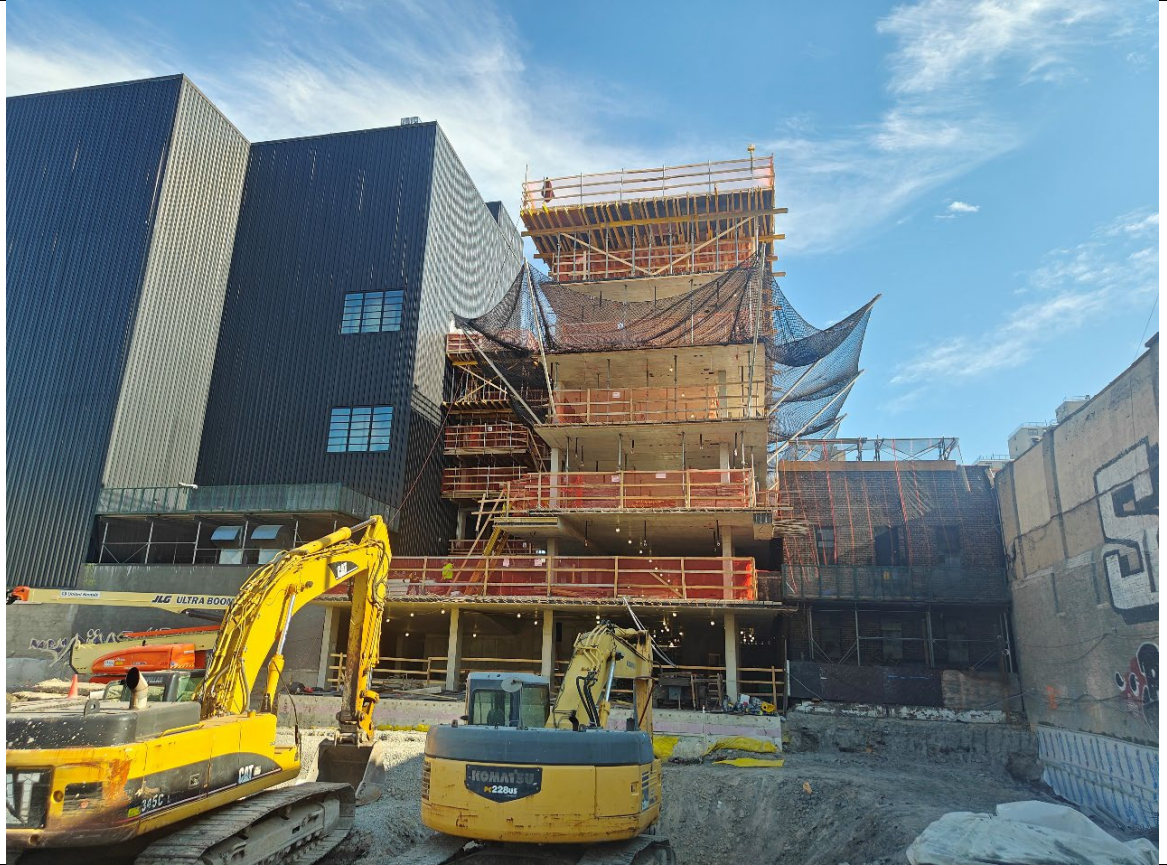
Photo 1- Representative view of the superstructure.
