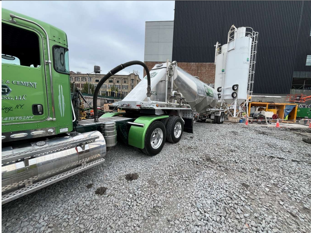
Photo 3- Representative photo of slag delivery.
