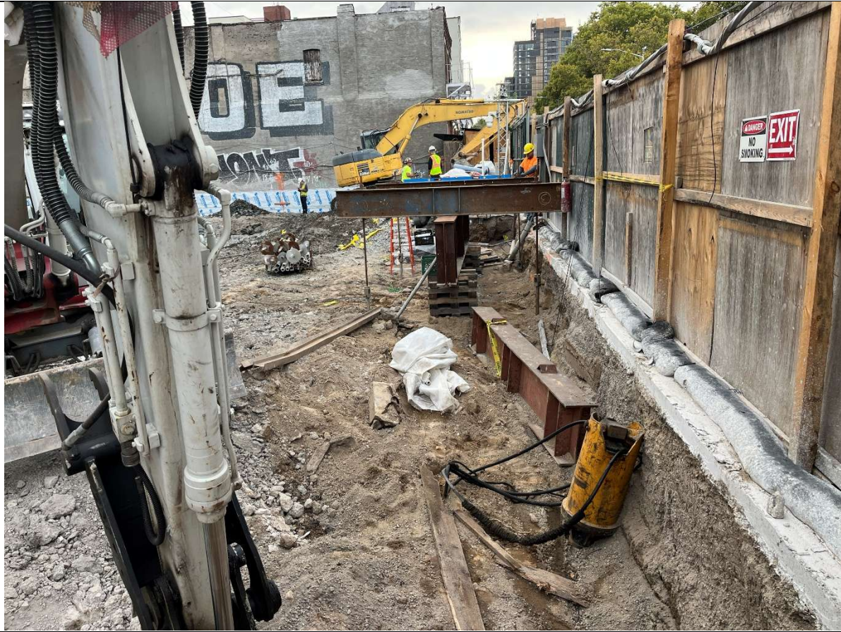
Photo 5- Representative photo of FSR helical pile load test.
