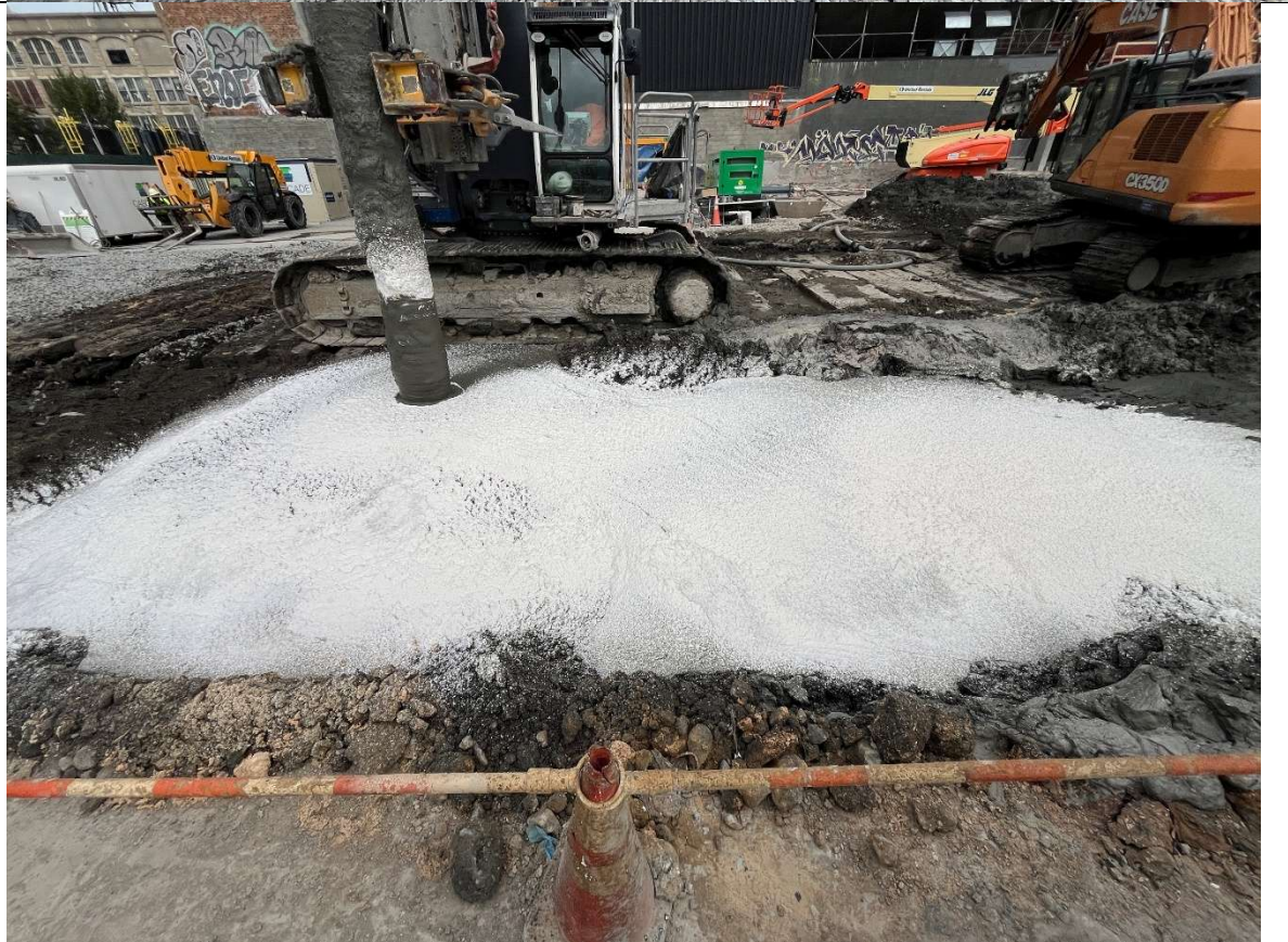
Photo 4- Representative photo of ISS Column installation.
