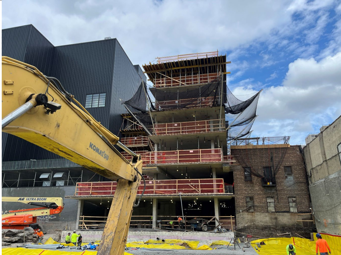
Photo 4- Representative photo of superstructure in the Butler Corridor.
