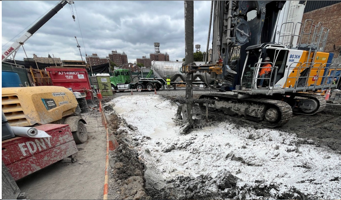
Photo 1- Representative photo of ATMOS foam applied to ISS drilling area.
