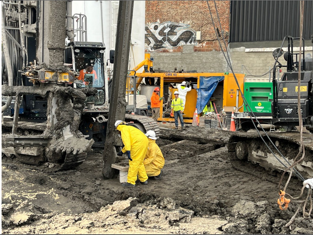
Photo 5- Representative photo of Cascade collecting a wet mix sample from Column 74 at 35'.
