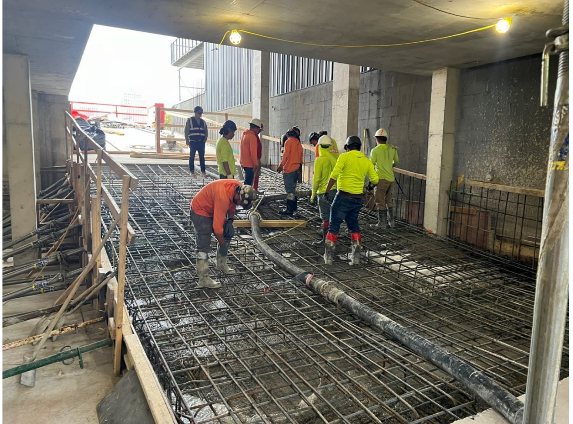
Photo 2- Representative photo of concrete being poured for a ramp.
