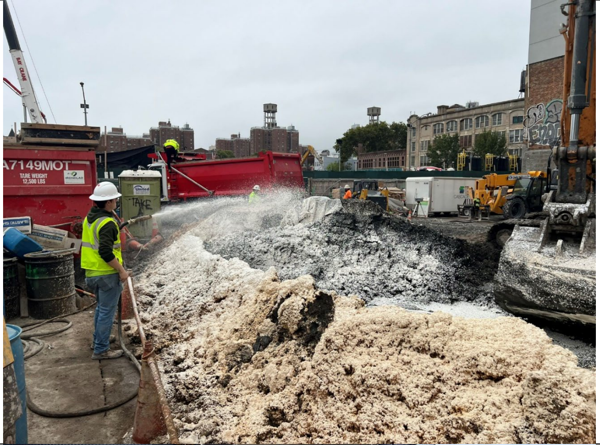
Photo 1- Representative photo of ATMOS foam applied to ISS drilling area.
