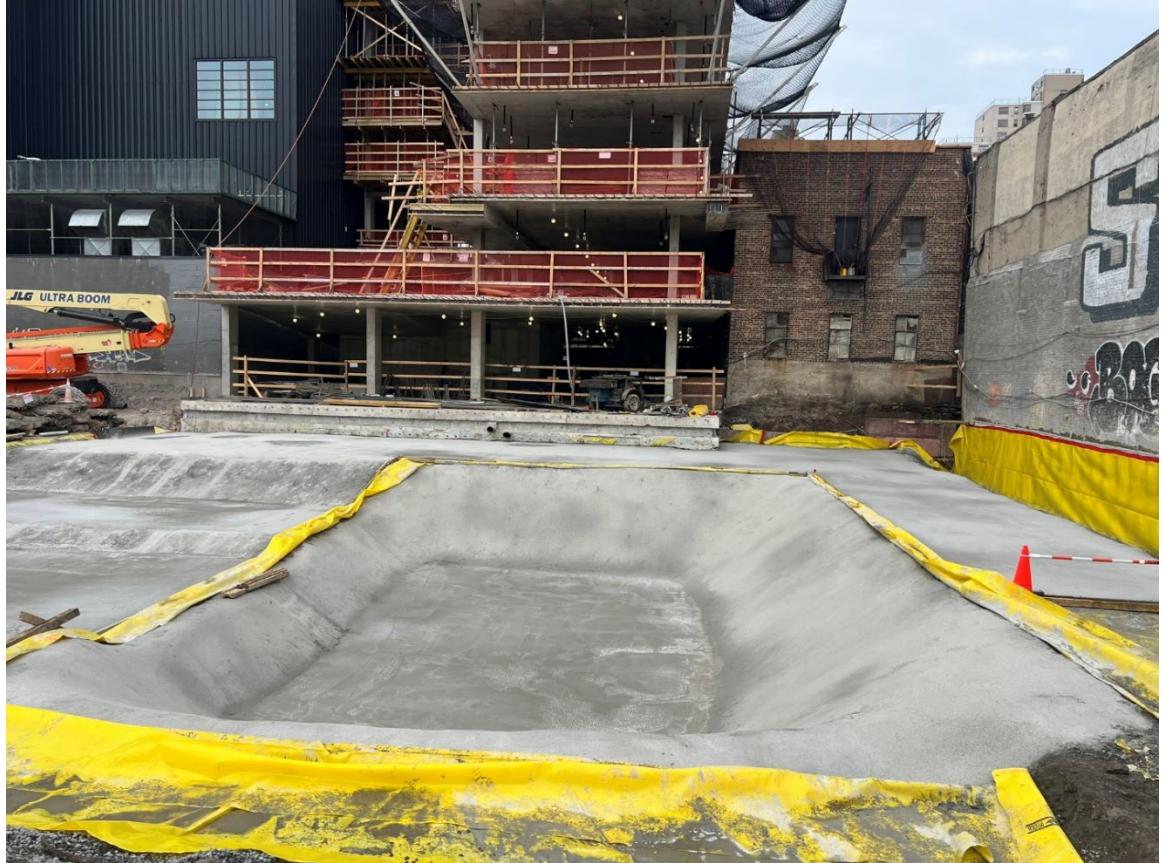
Photo 2- Representative photo of rat slab poured.
