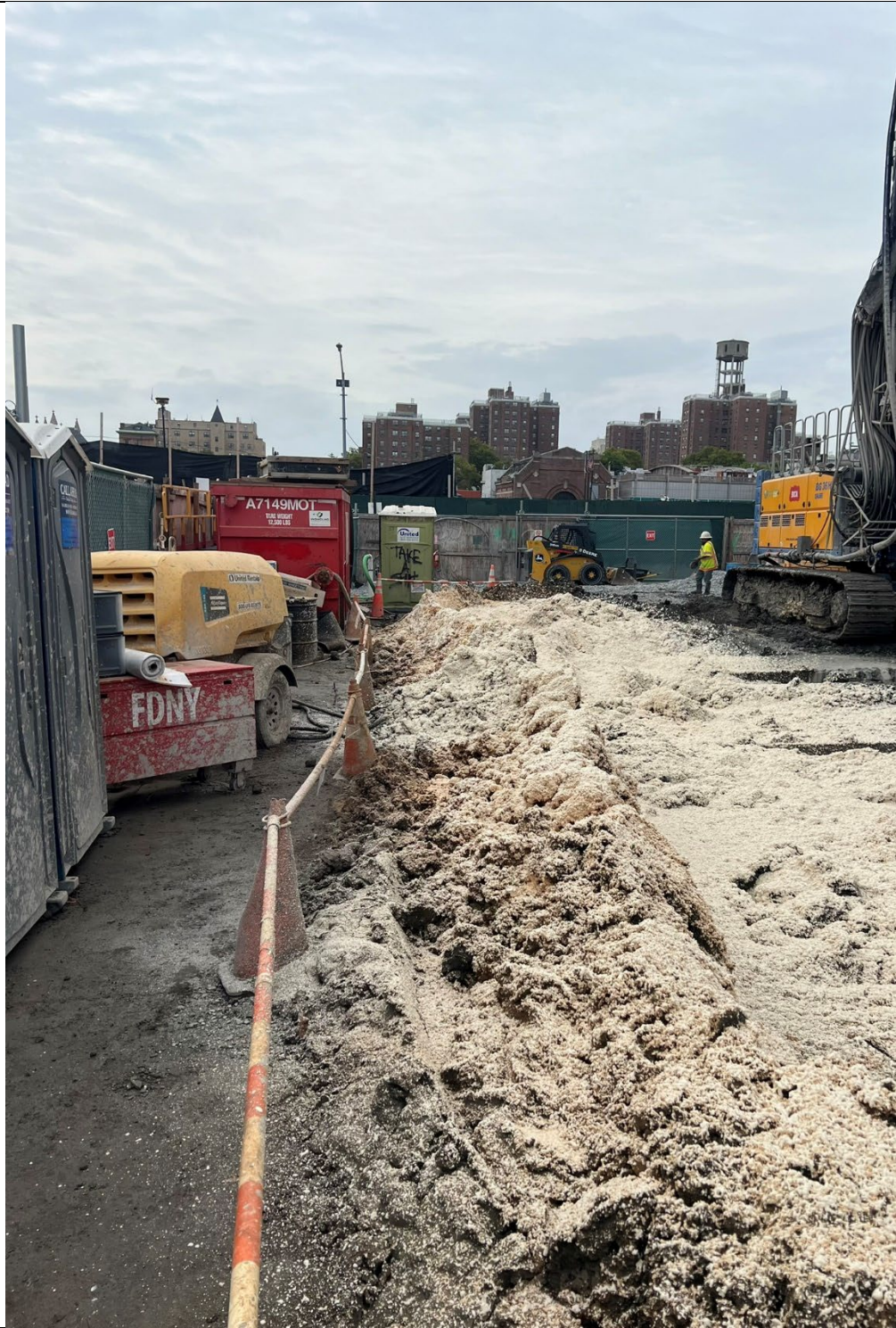
Photo 5- Representative photo of the work area sprayed with ATMOS foam at the end of the day.
