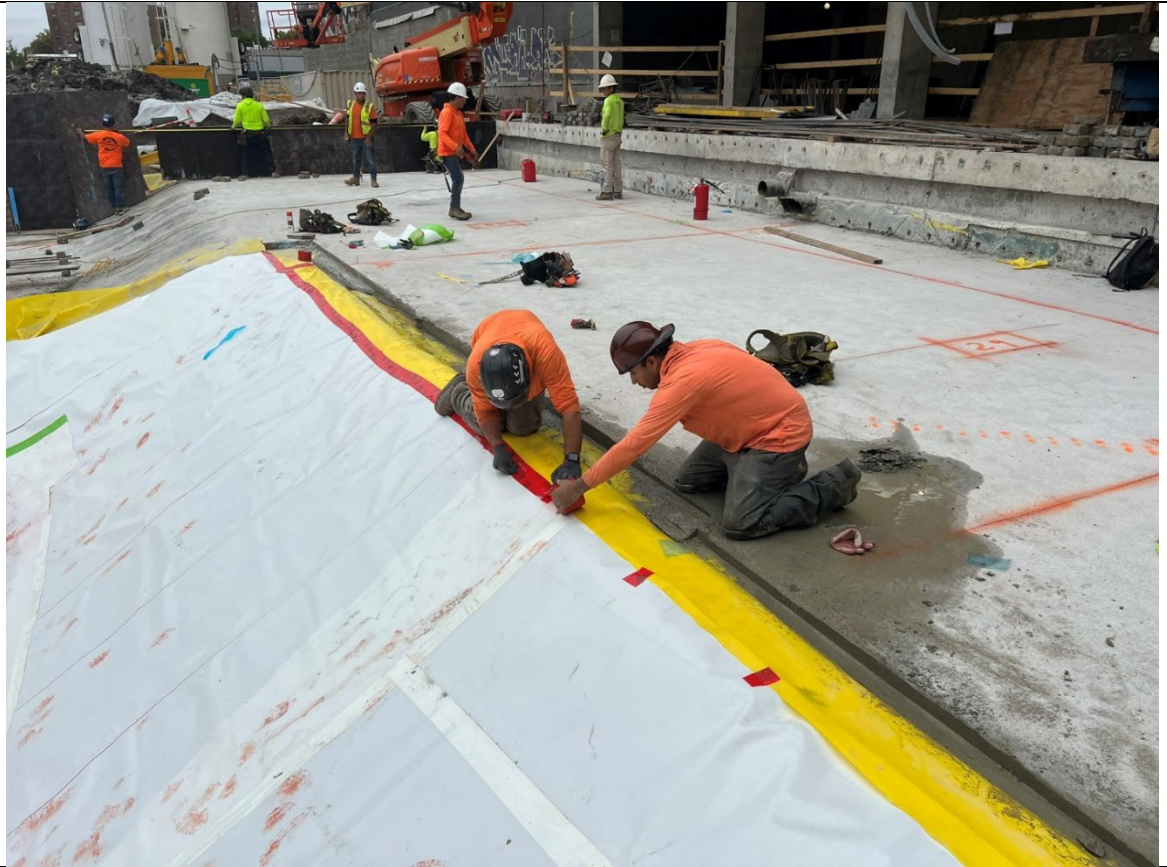
Photo 3- Representative photo of tying in the waterproofing with the vapor barrier.
