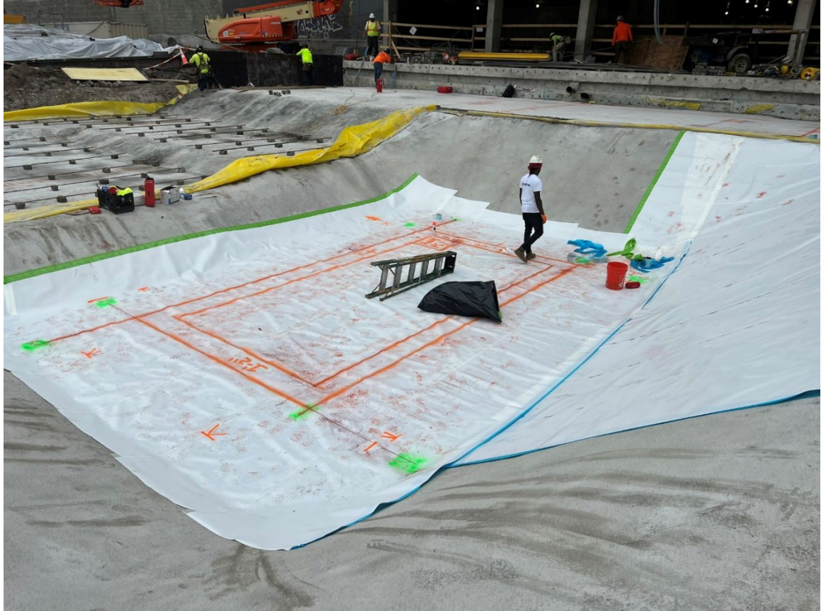
Photo 2- Representative photo of water proofing being applied to the elevator pit.
