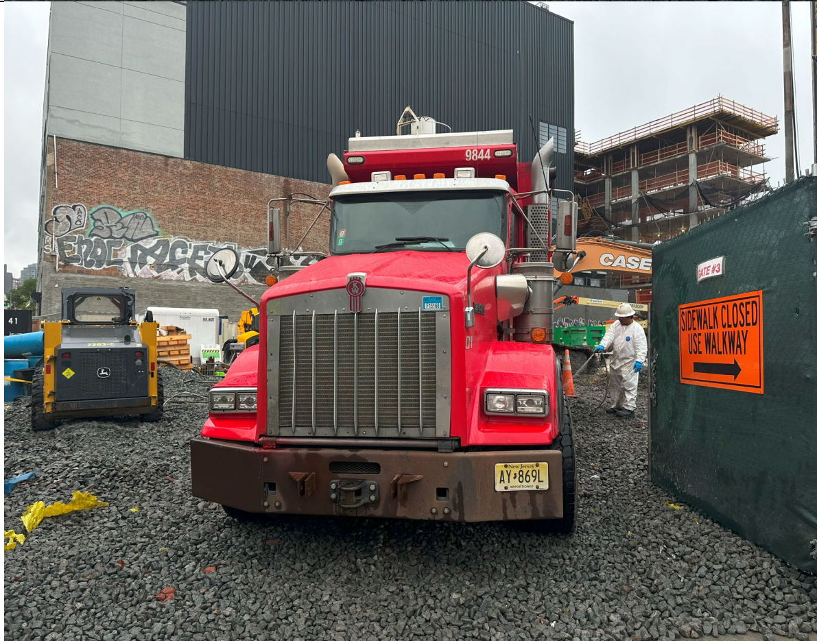
Photo 2- Representative view of truck tires being wash before exiting site.
