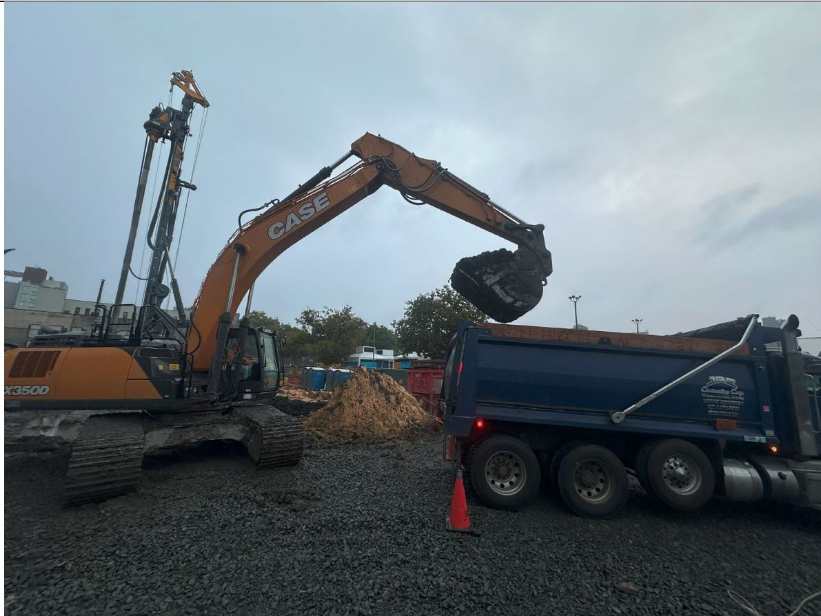
Photo 1- Representative view of truck being load.
