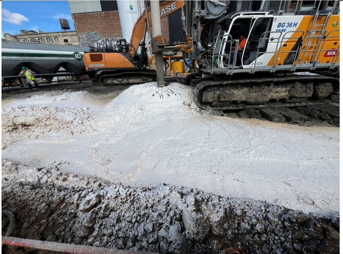
Photo 1- Representative photo of ATMOS foam applied during ISS column installation.
