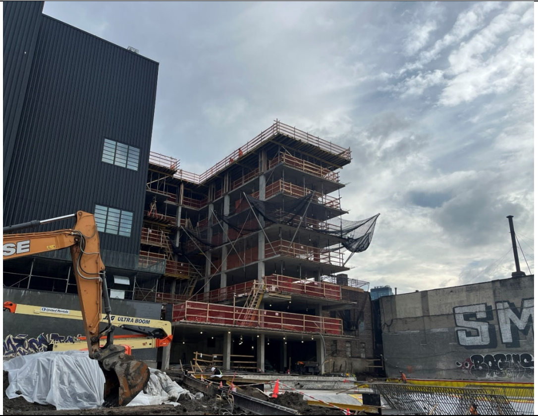
Photo 5- Representative photo of superstructure in the Butler Corridor.
