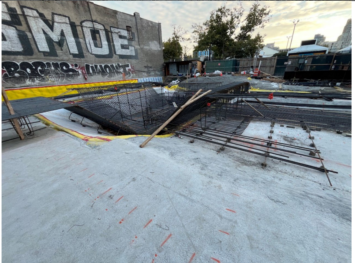
Photo 2- Representative photo of rebar installed over rat slab.
