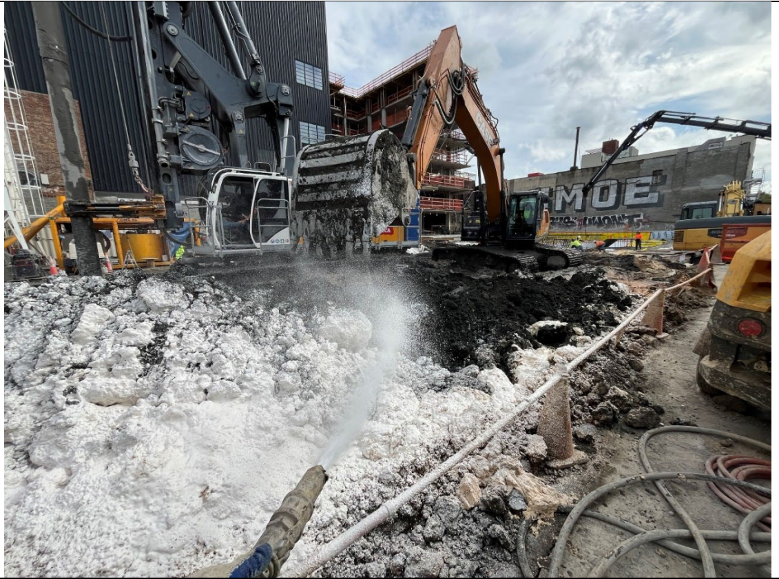
Photo 5- Representative photo of ATMOS foam application during stockpile relocation.
