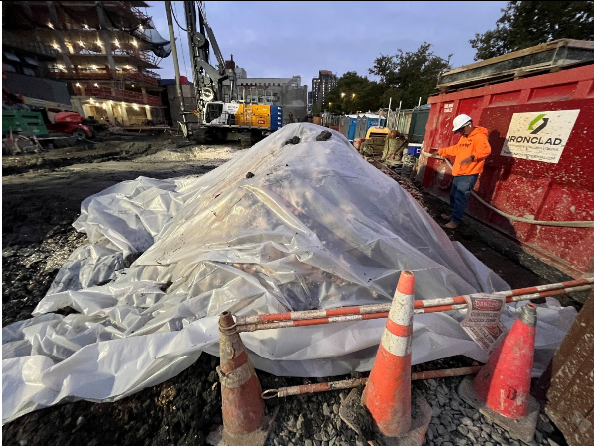
Photo 5- Representative photo of swell stockpile covered with poly at the end site activities.
