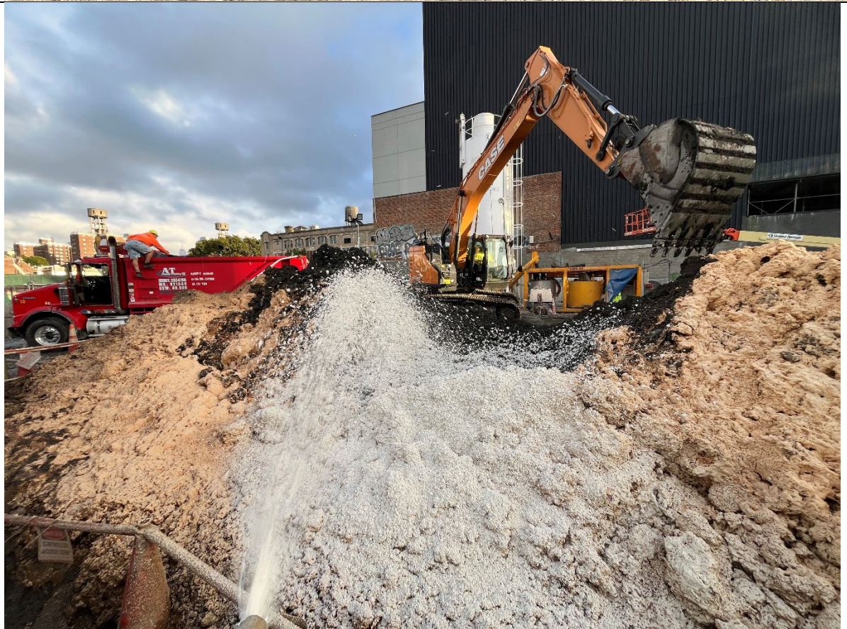
Photo 2- Representative photo of ATMOS foam application during swell loadout.
