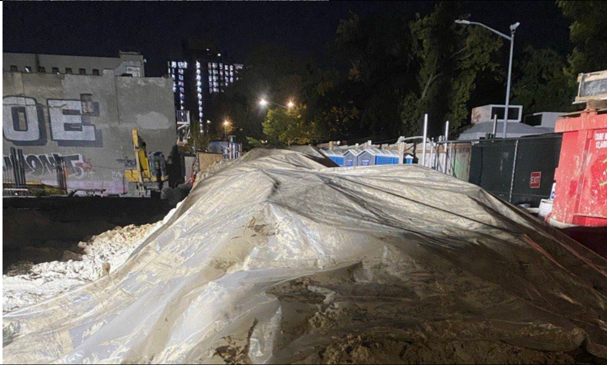
Photo 4- Representative photo of swell material covered with ATMOS foam at the end of site activities and covered in poly.
