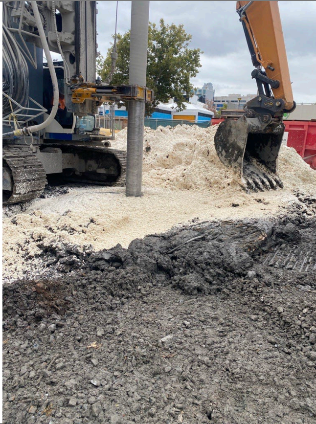
Photo 3- Representative photo of ISS column installation.
