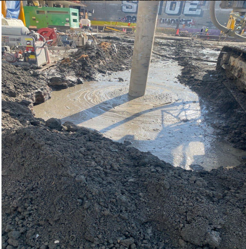
Photo 2- Representative photo of ISS column installation.
