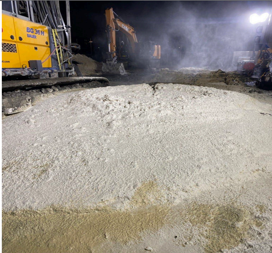
Photo 3- Representative photo of swell material covered with ATMOS foam.
