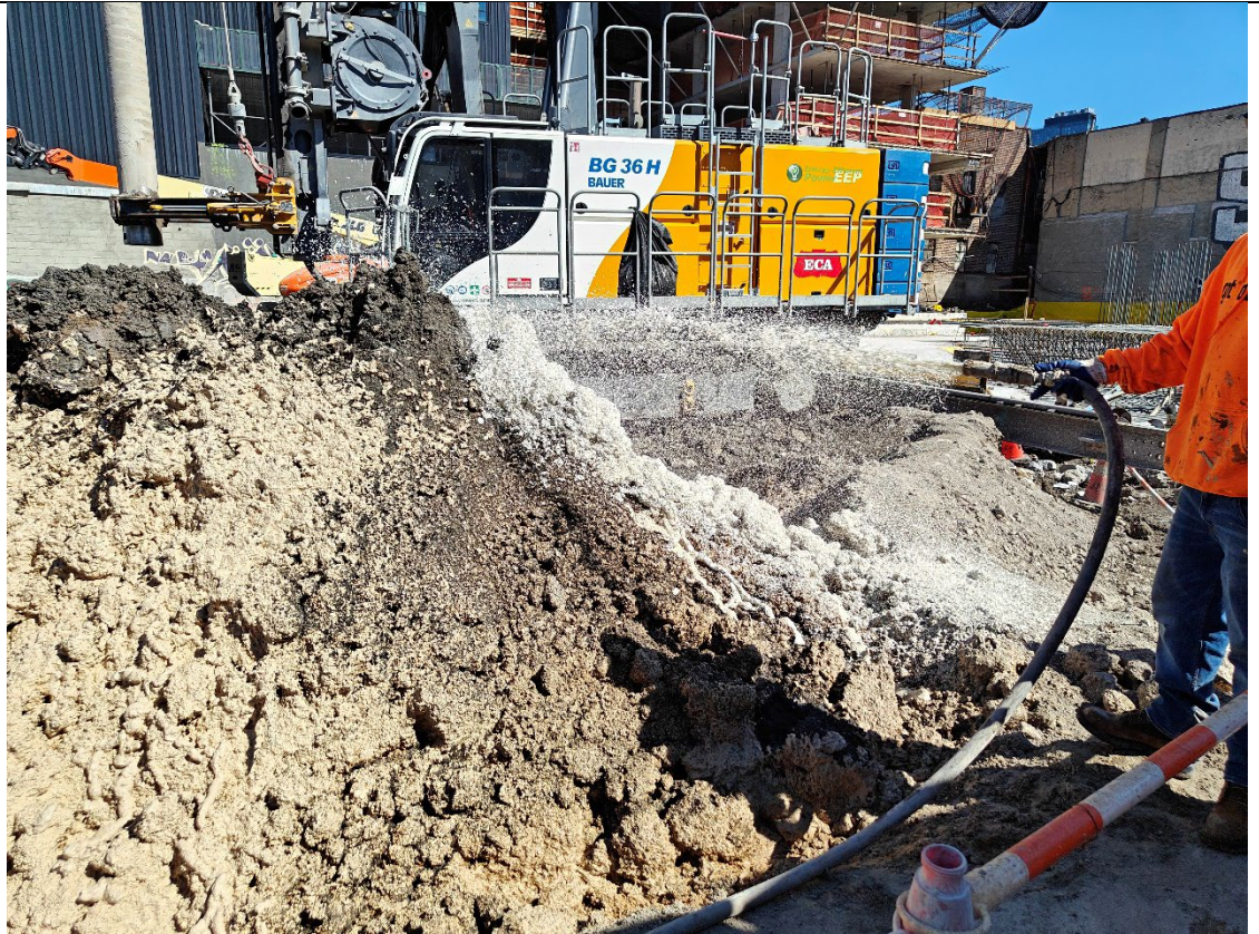
Photo 3- Representative view of ATMOS application to swell stockpile.
