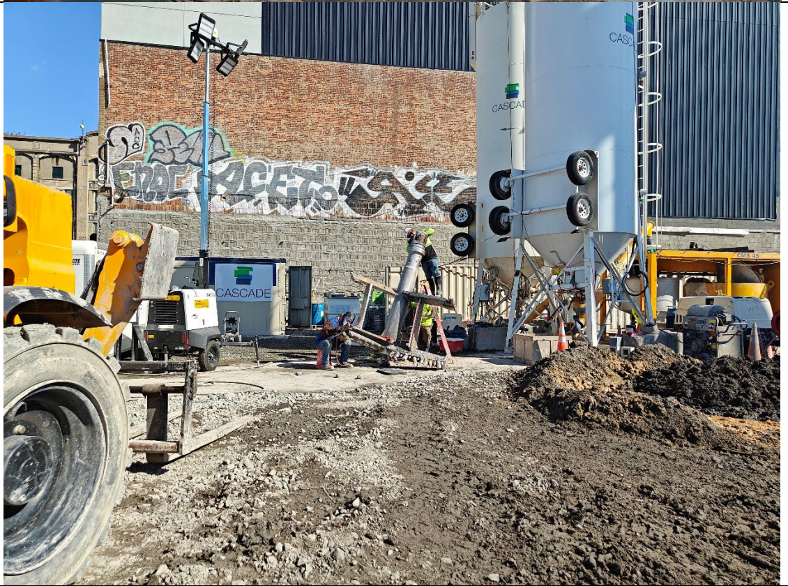
Photo 2- Representative photo of augur maintenance.
