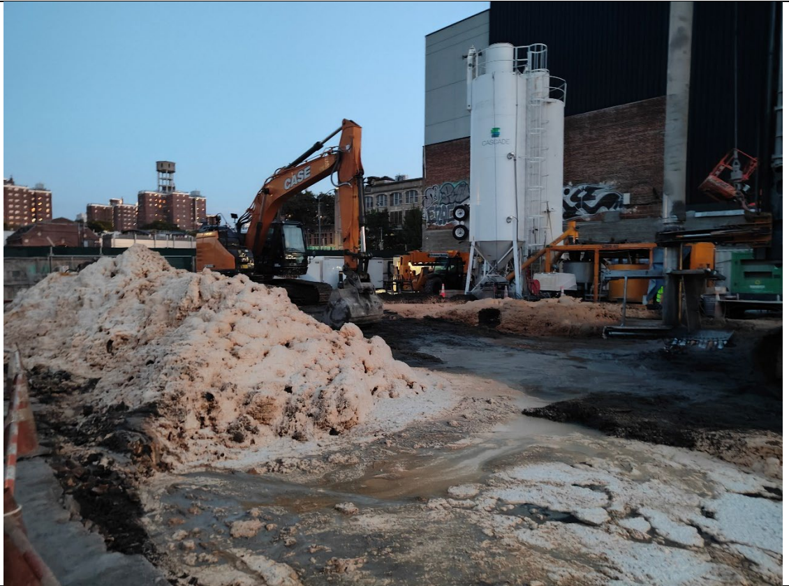
Photo 1- Site at the start of the day's activities.
