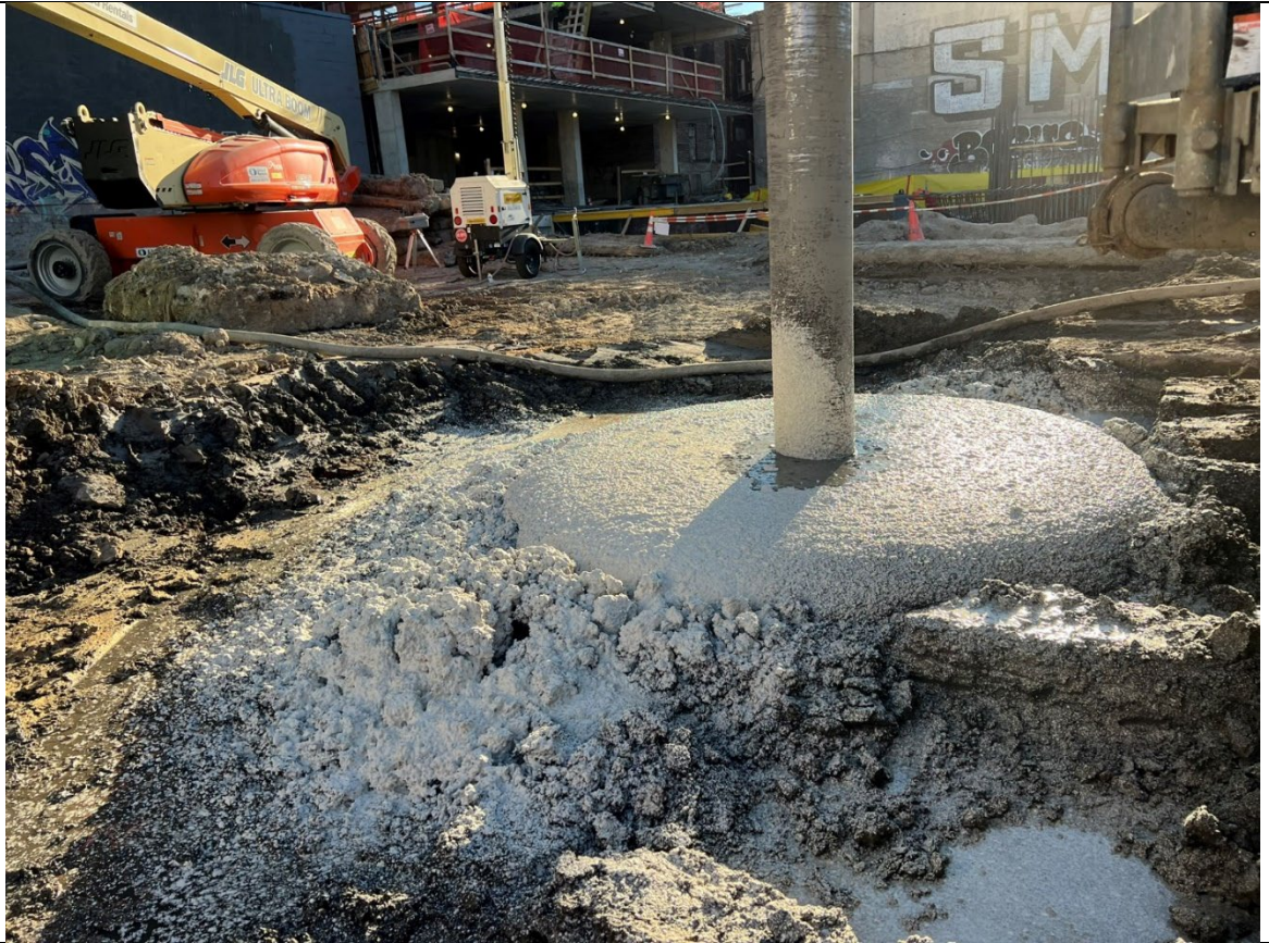
Photo 1- Representative photo of drilling an ISS column.
