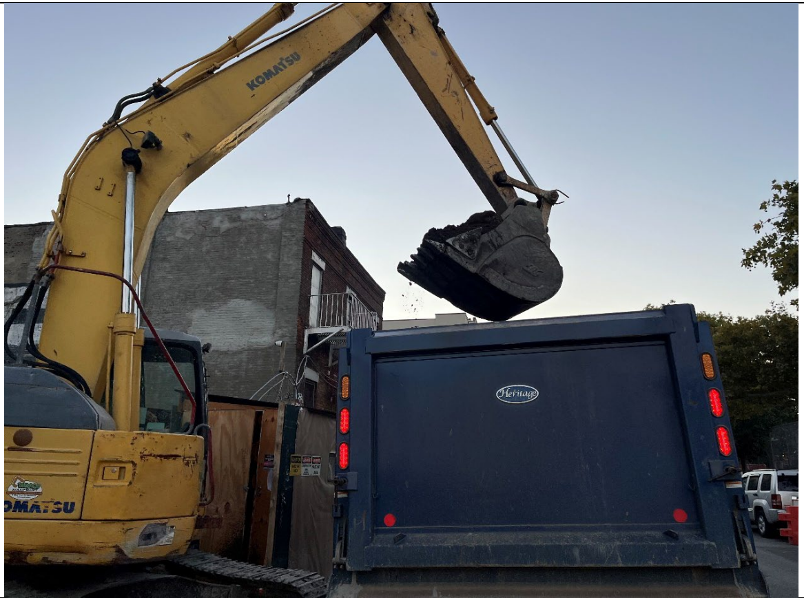
Photo 1- Representative photo of loading truck with swell material.
