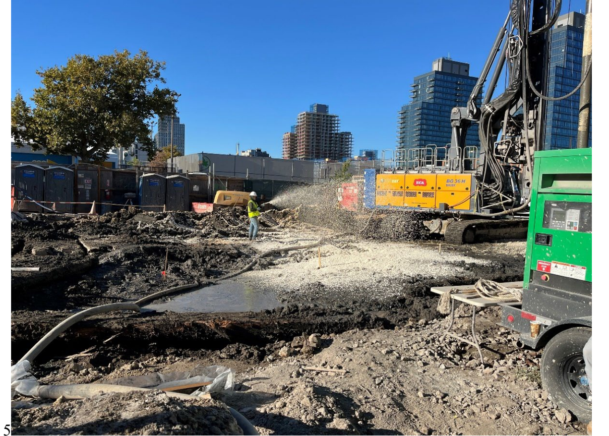
Photo 4- Representative photo of ATMOS foam sprayed over work area.
