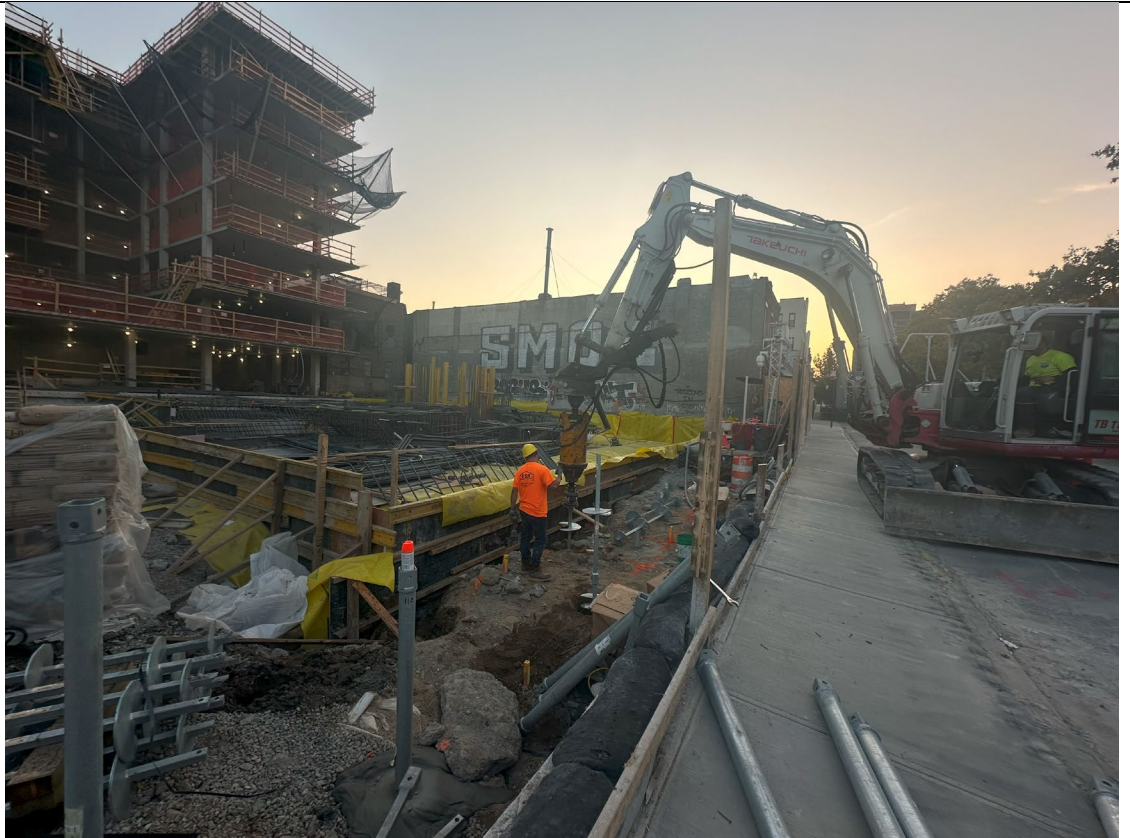
Photo 1- Representative photo of FSR performing Helical pile installation.
