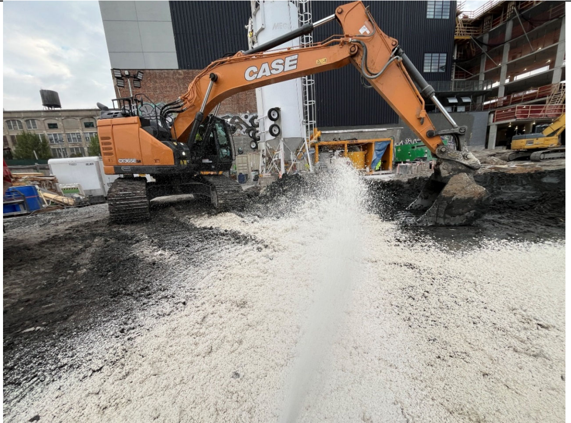
Photo 1- Representative photo of ATMOS application to swell material being loaded out.
