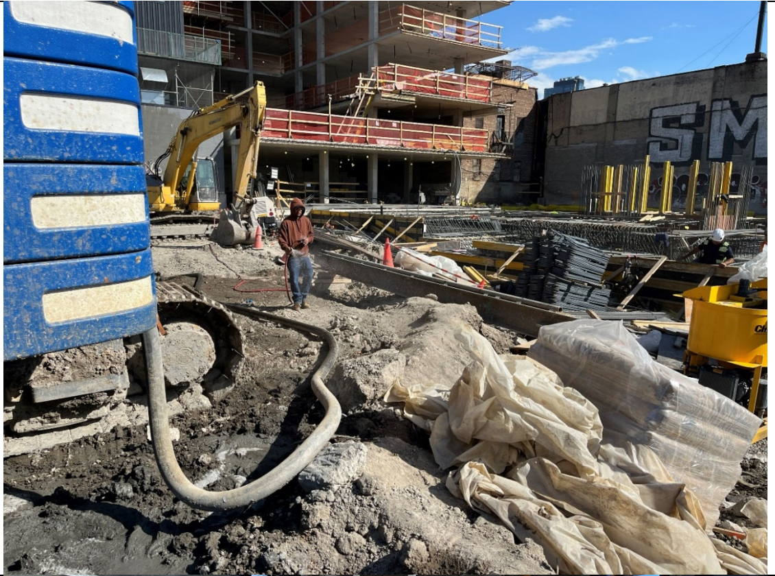
Photo 3- Representative view of laborer utilizing water to suppress dust.
