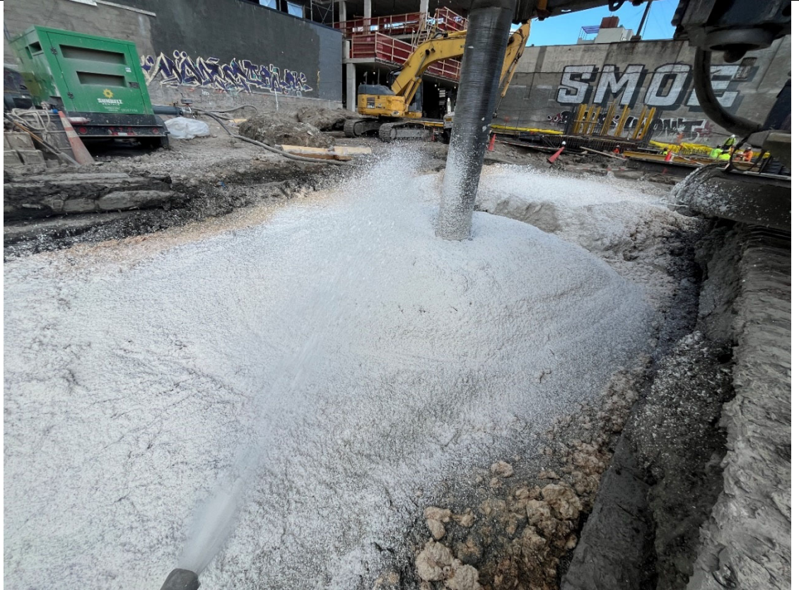
Photo 4- Representative photo of ATMOS application during ISS column installation.
