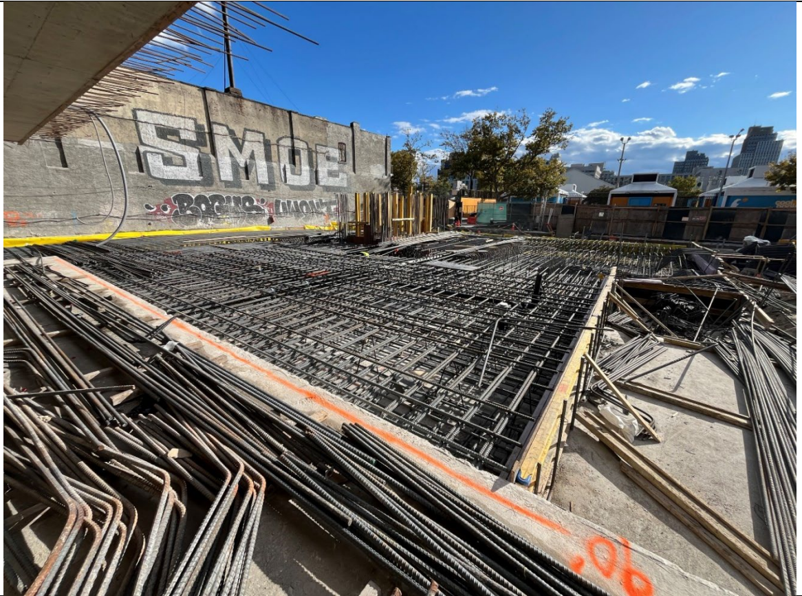
Photo 3- Representative view of rebar installed by concrete courses.
