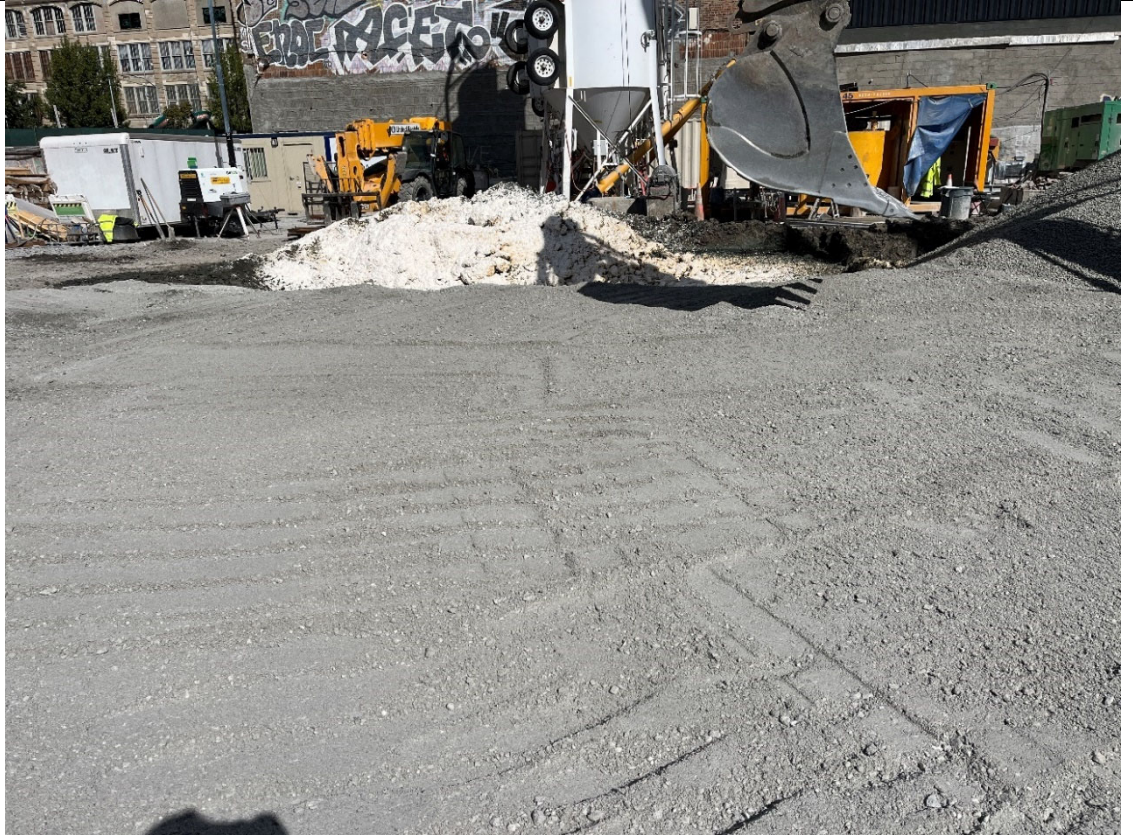
Photo 4- Representative photo of graded ISS area.
