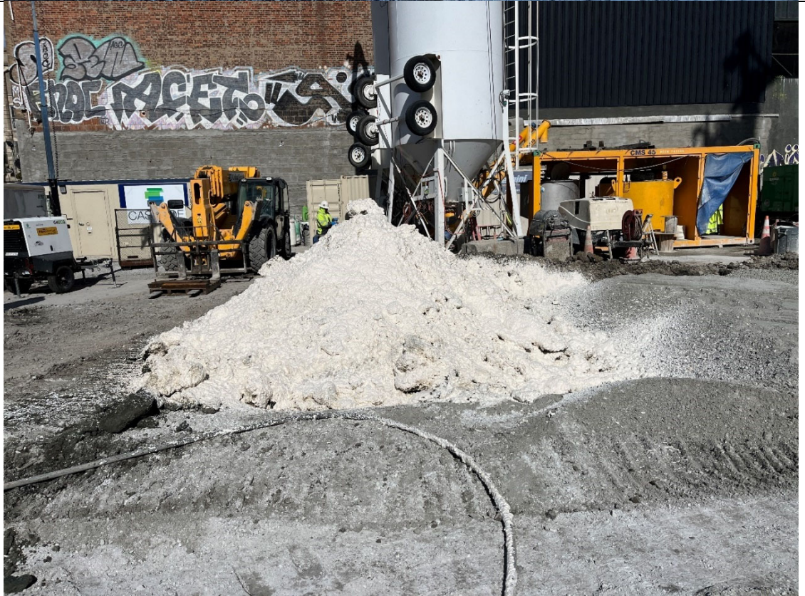
Photo 2- Representative photo of swell stockpile covered in ATMOS foam at the end of site activities.
