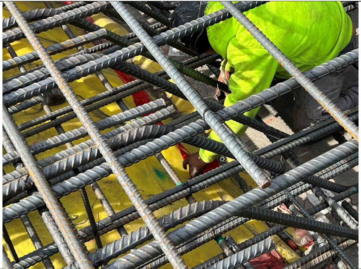
Photo 5- Representative photo of concrete courses repairing perforations in the vapor barrier.
