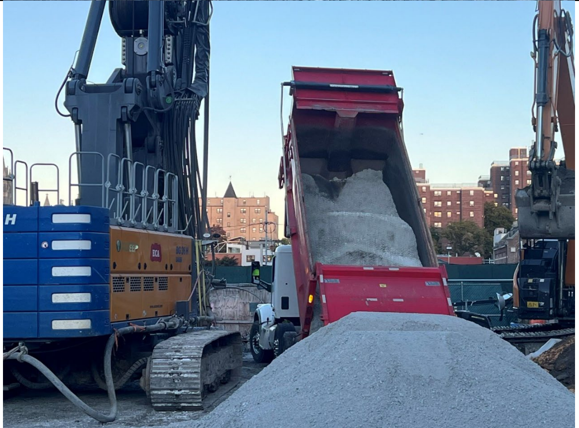
Photo 4- Representative photo of approved backfill being delivered.
