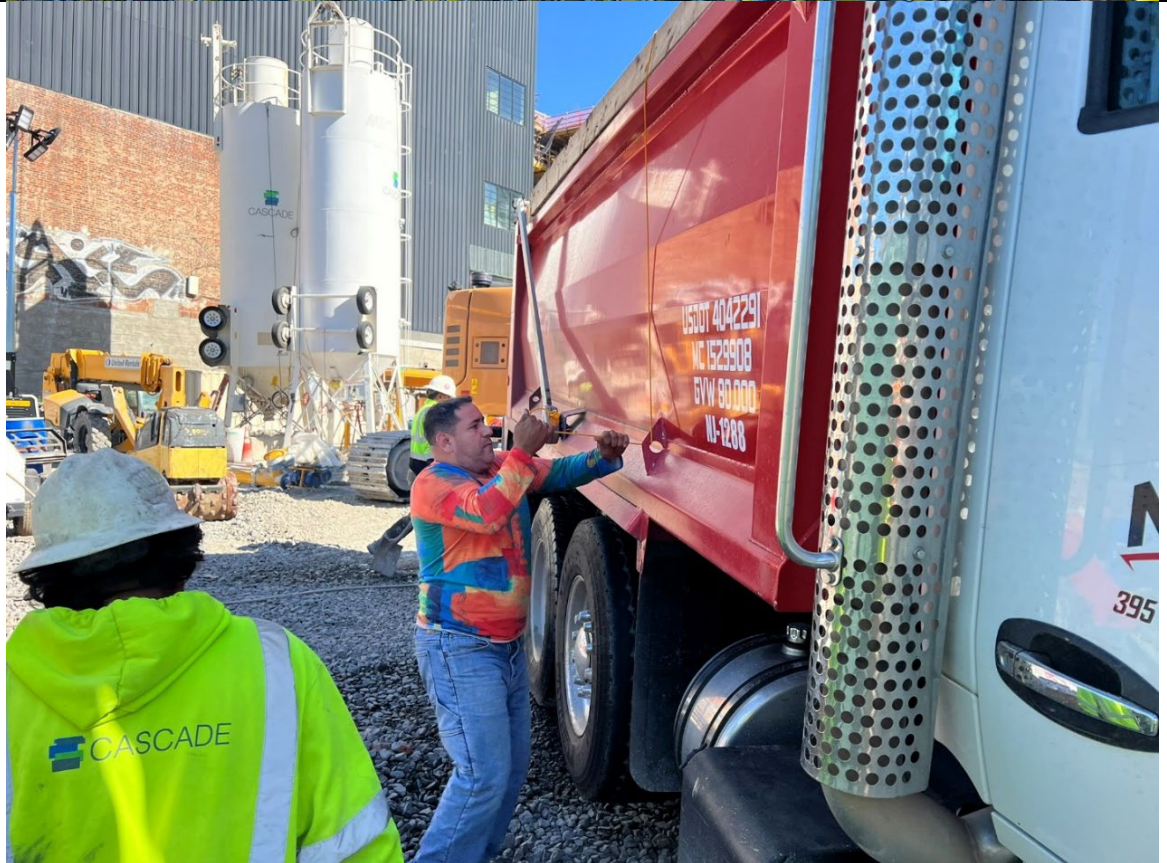
Photo 2- Representative photo of tying down the side of a truck properly prior to it exiting the Site.
