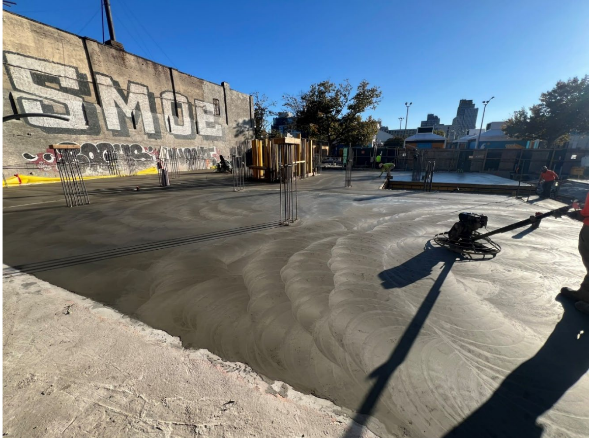
Photo 4- Representative photo of finishing concrete pour for the day.
