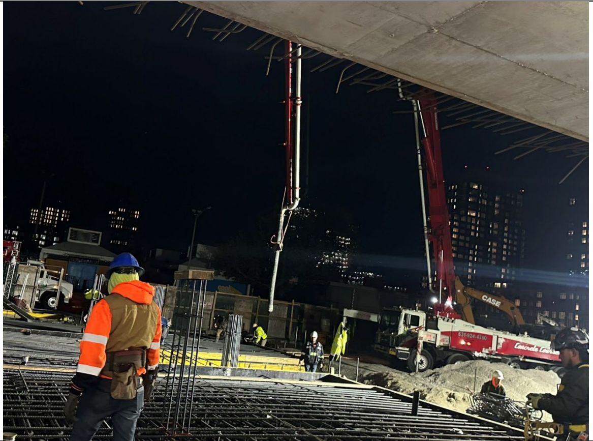
Photo 1- Representative photo of the pump truck on Site.
