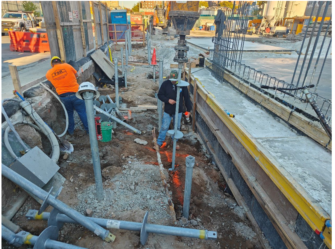
Photo 2- Representative photo of helical pile installation.
