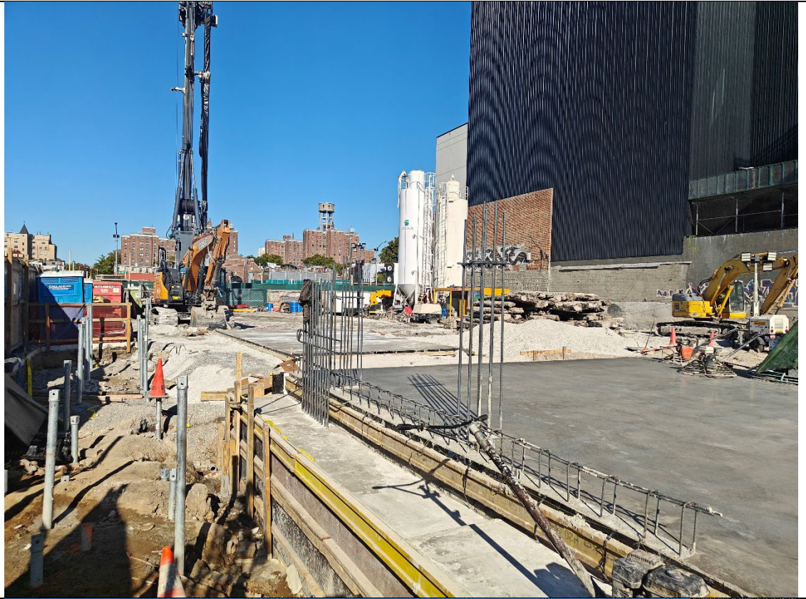
Photo 3- Representative photo of site at the end of the days activities.
