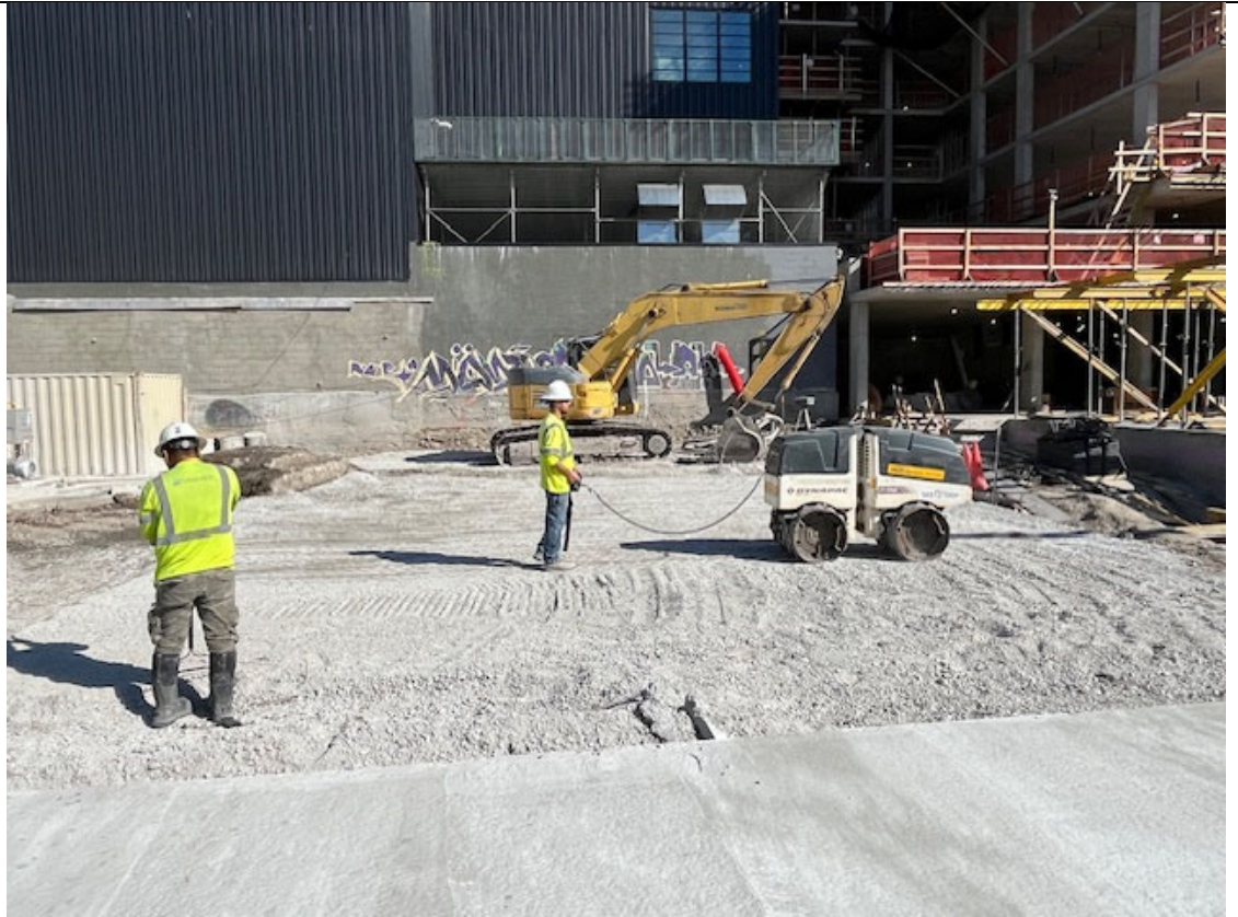
Photo 3- Representative photo of compacting limestone.
