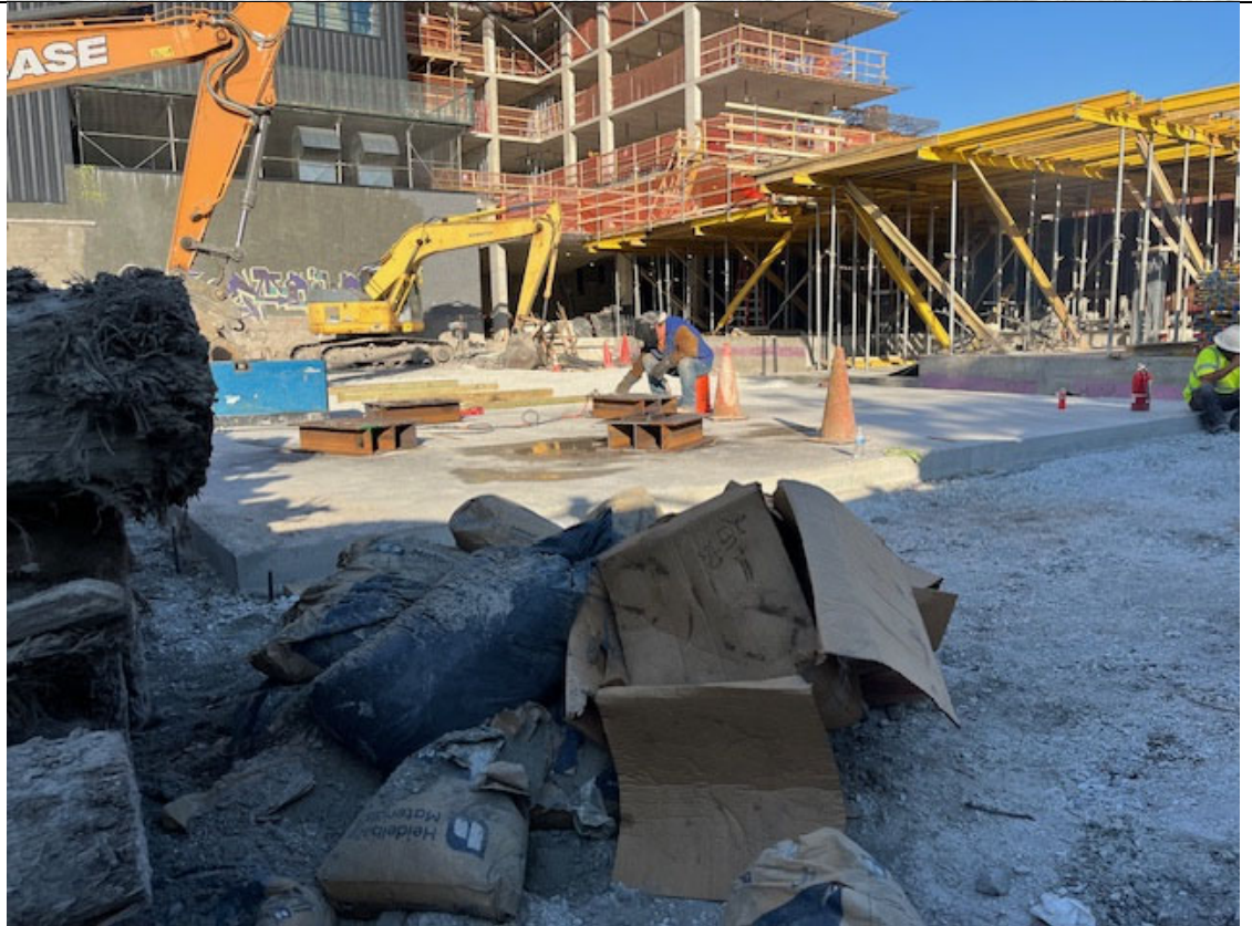
Photo 4- Representative photo of welding steel.
