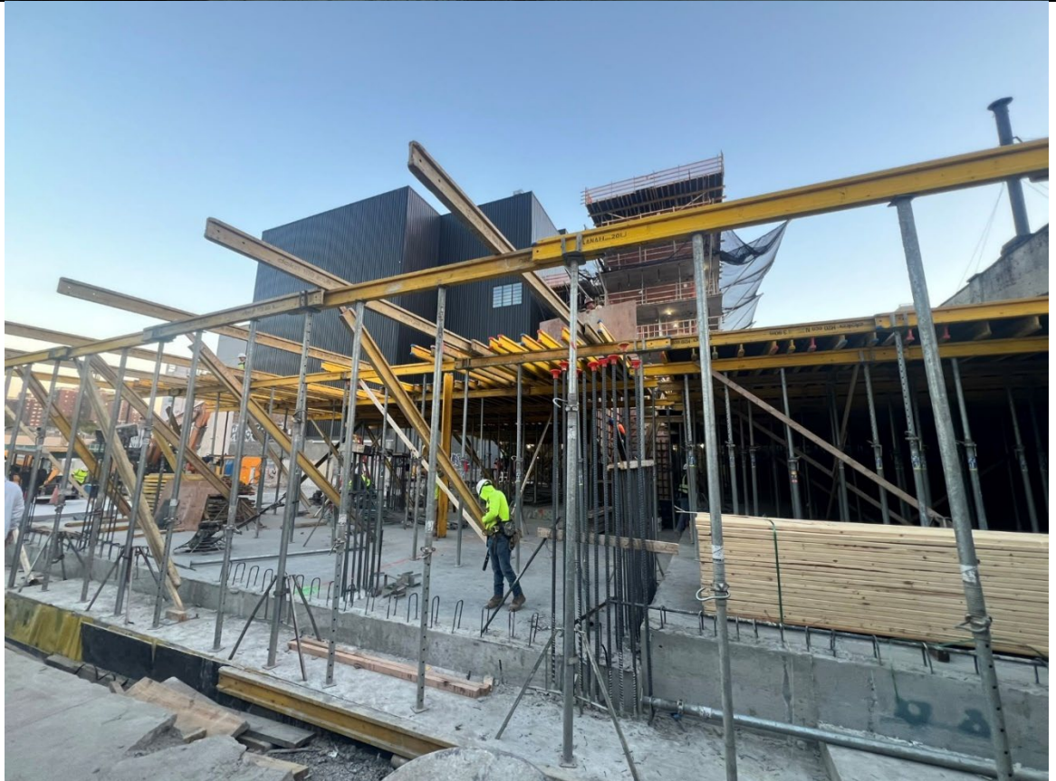
Photo 2- Representative photo of superstructure work in phase 2.
