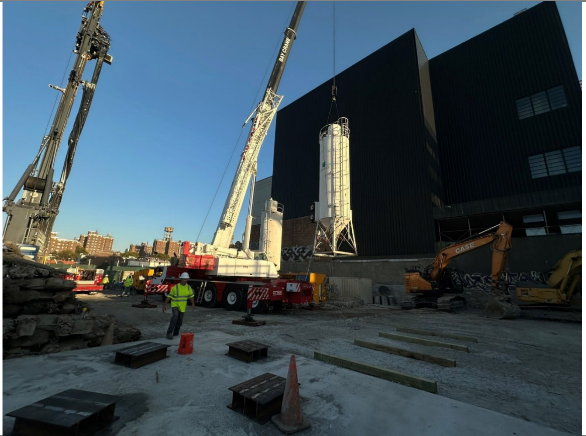
Photo 1- Representative photo of ISS equipment being moved.
