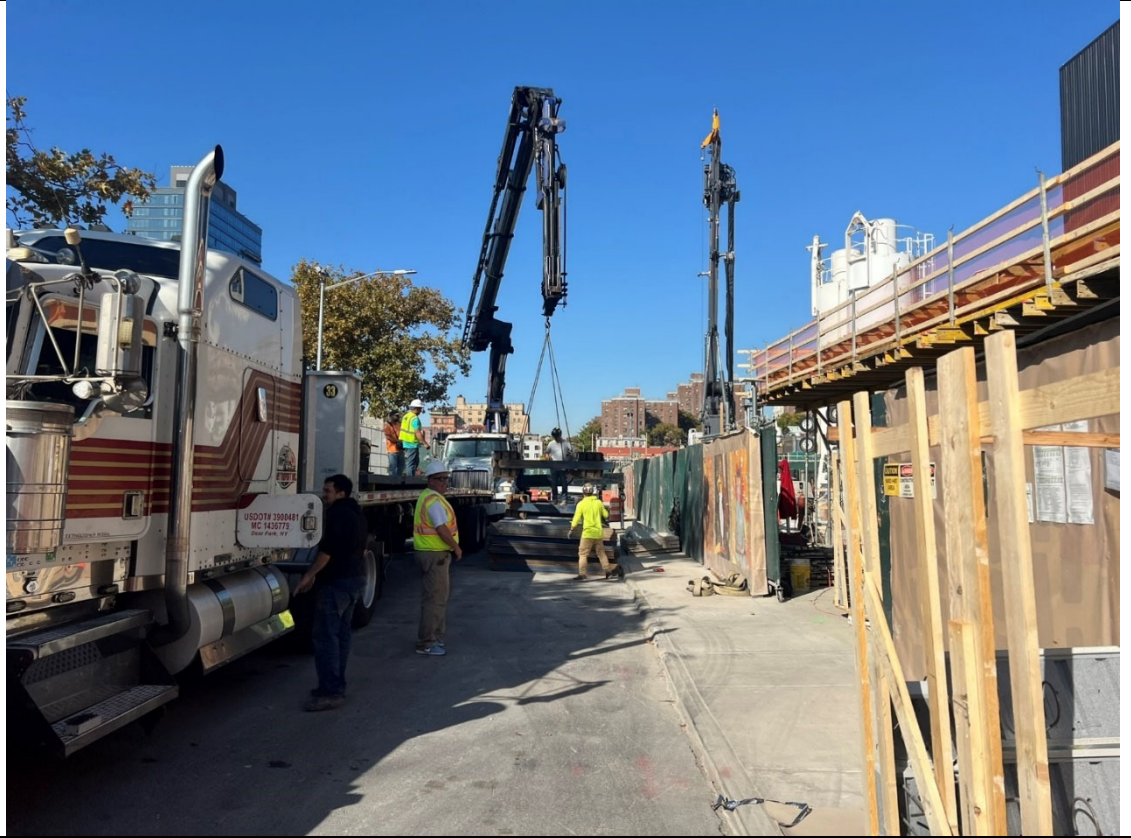
Photo 3- Representative photo of the delivery of a shoring box.
