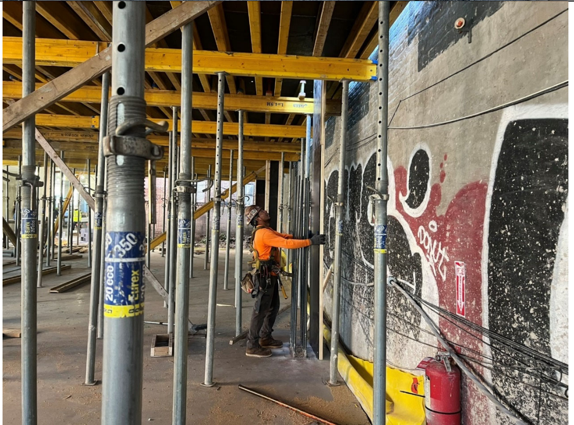
Photo 2- Representative photo of superstructure work in phase 2.
