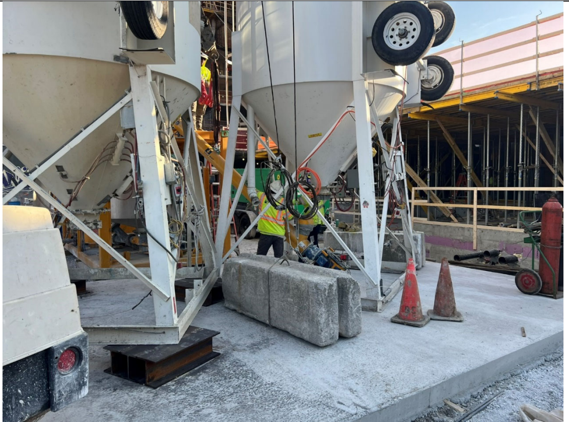
Photo 1- Representative photo of Cascade connecting equipment to resume drilling ISS columns.
