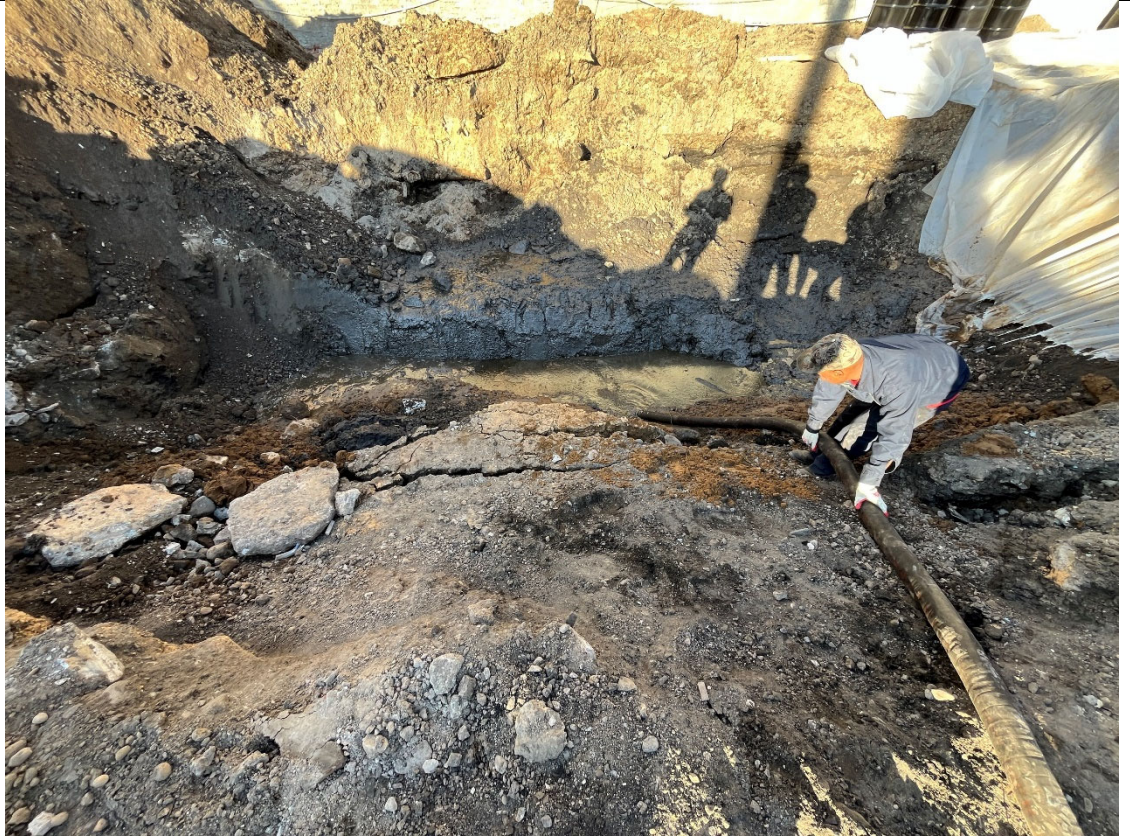
Photo 1- ABC Tank pumps out water from 10,000 gallon tank grave.
