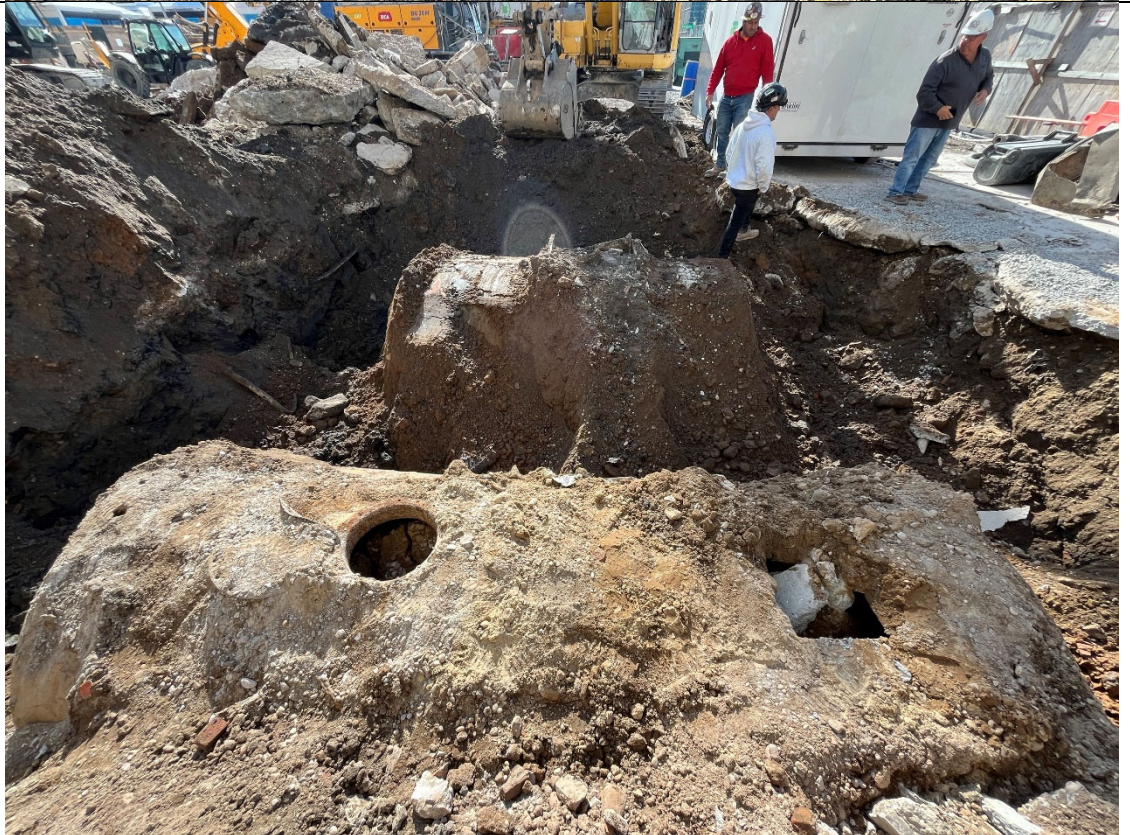
Photo 2- Representative photo of exposure of the two smaller tanks.
