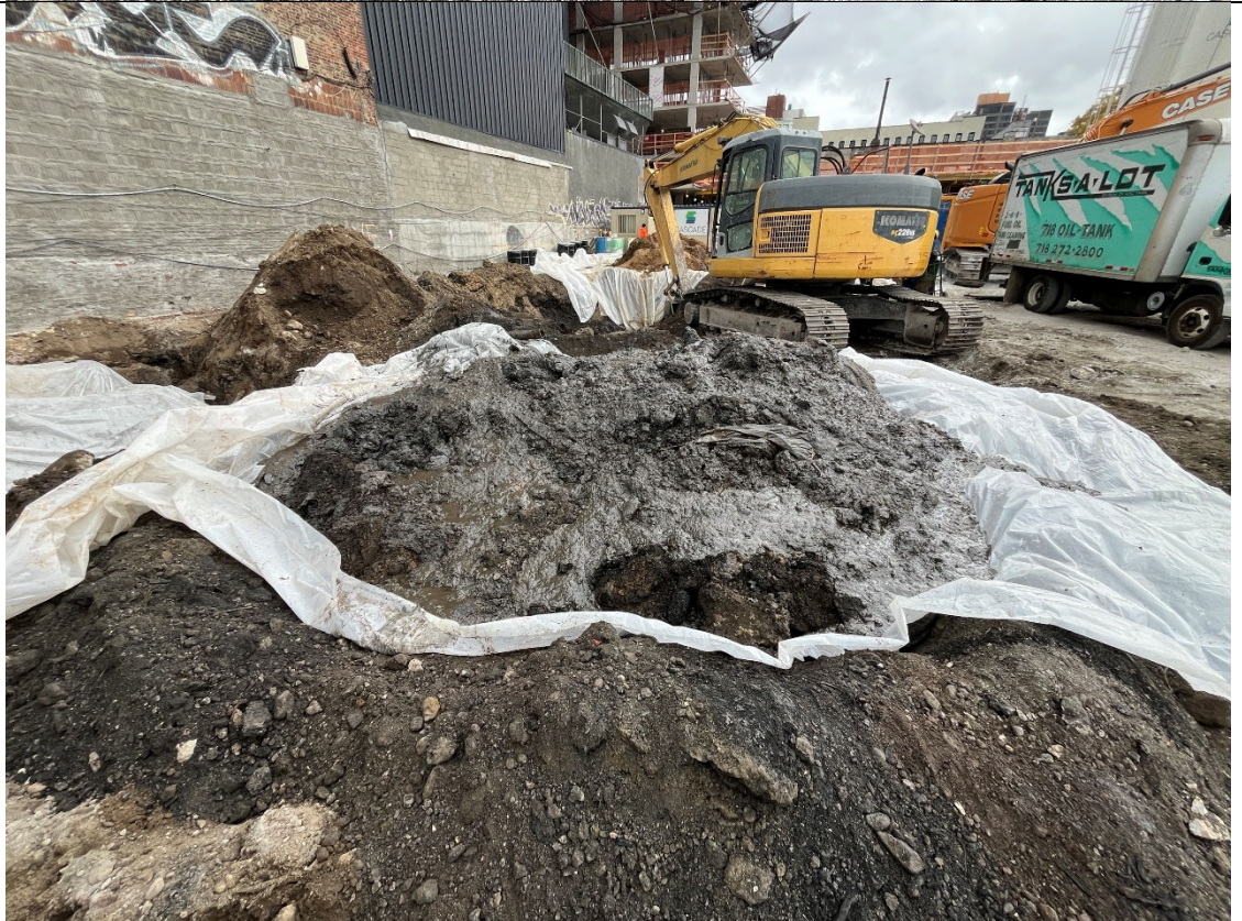
Photo 2- Representative photo of excavation of grossly contaminated material from the 10,000-gallon tank grave.
