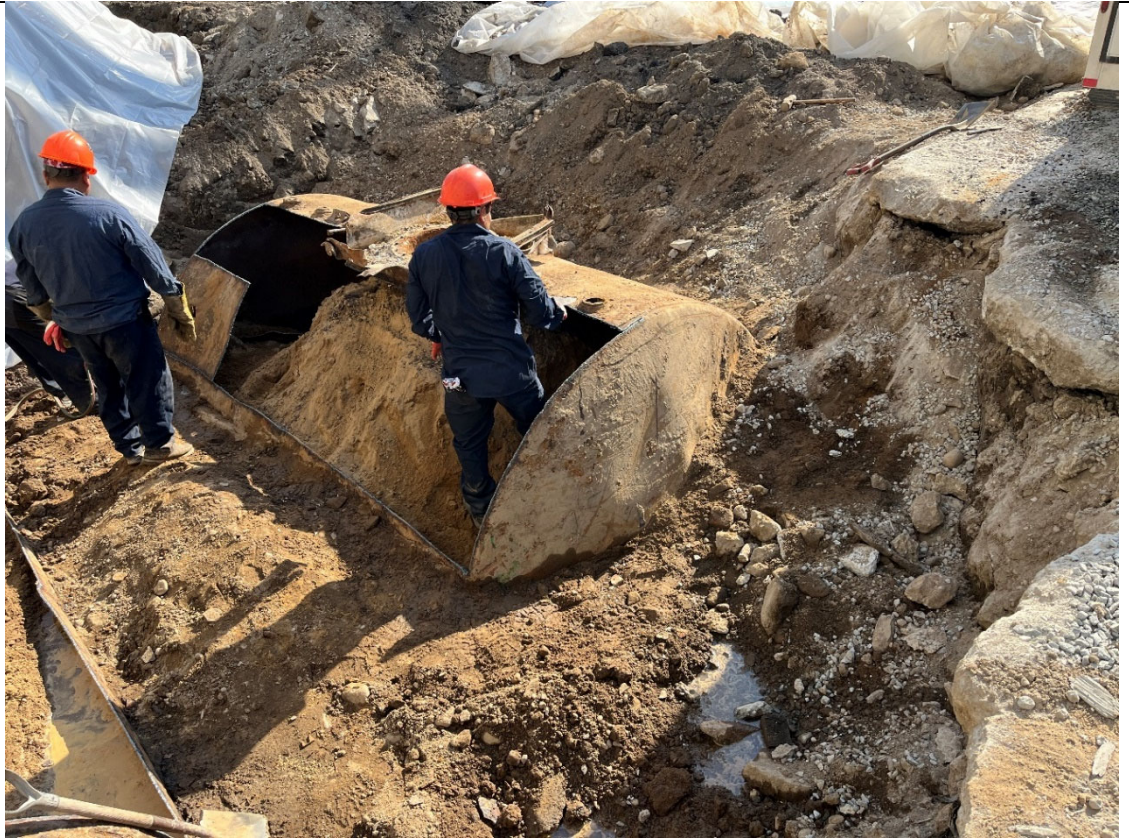
Photo 1- ABC Tank Repair cutting open the smaller UST in the northwest portion of the site.
