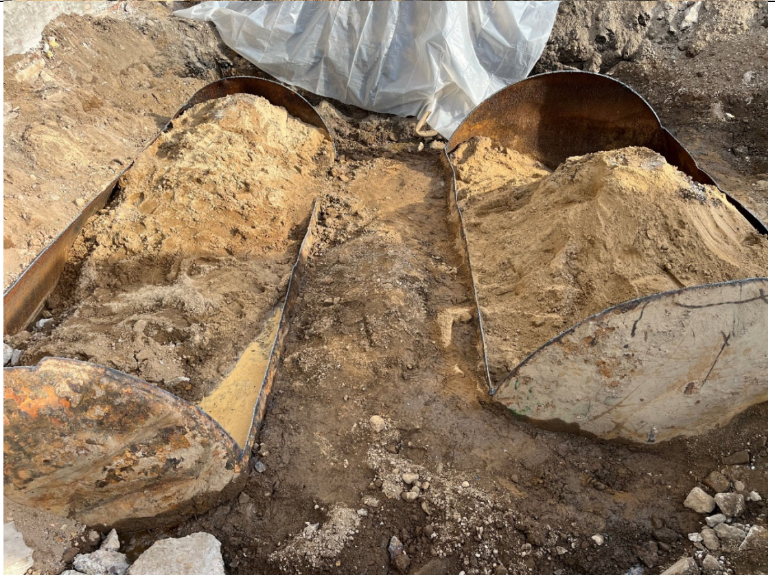
Photo 2- Representative photo of the contents of the two USTs in the northwest portion of the site.
