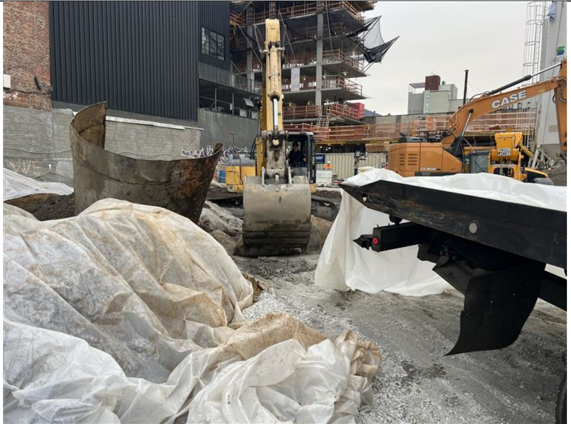
Photo 1- ABC Tank Repair cutting tank to be removed offsite.
