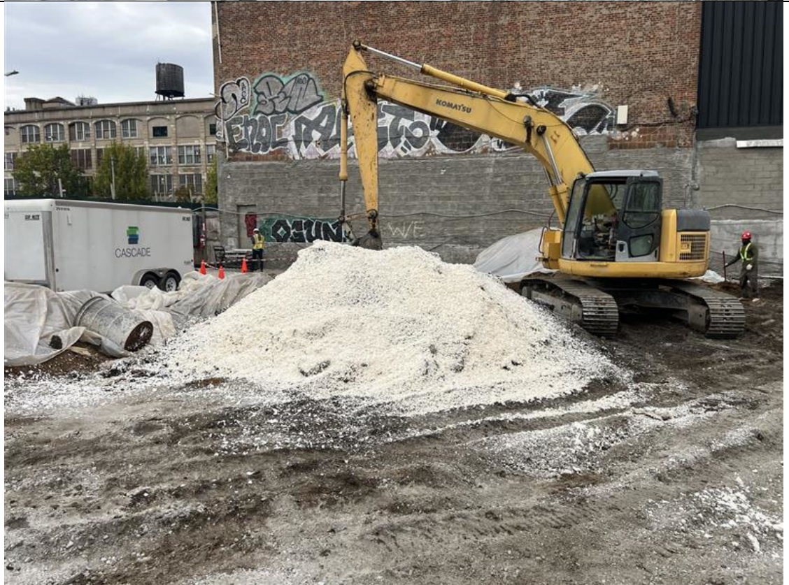
Photo 2- Representative photo of tank stockpile covered with Atmos foam.
