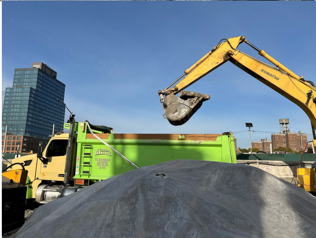
Photo 4- Representative photo of concrete trucking.
