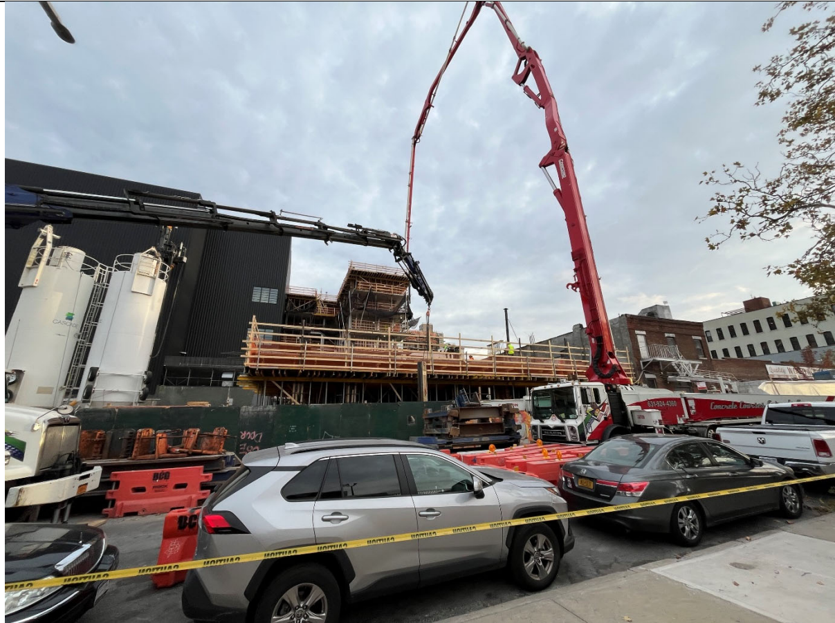
Photo 1- Concrete Courses pouring the second floor of the Phase II Superstructure.
