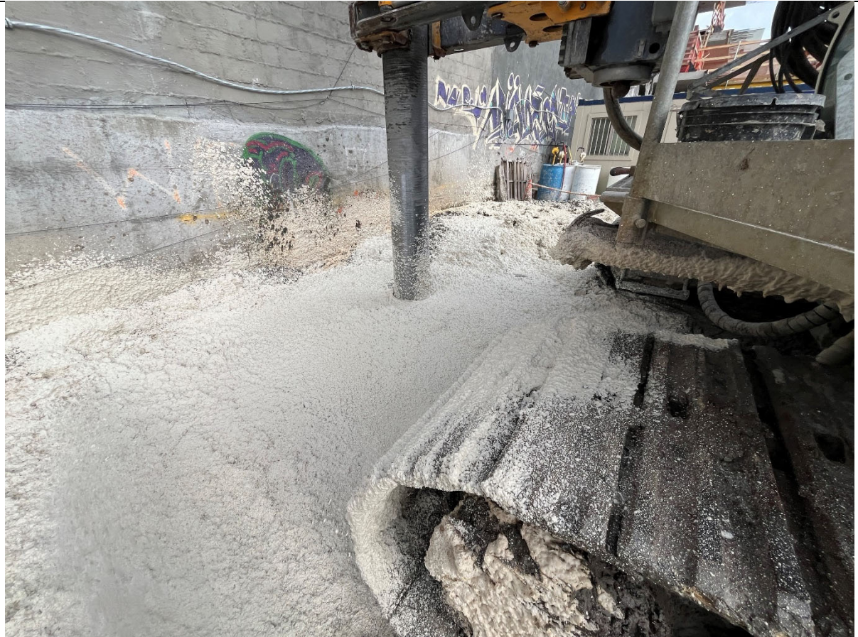
Photo 3- Representative photo of ISS column installation.
