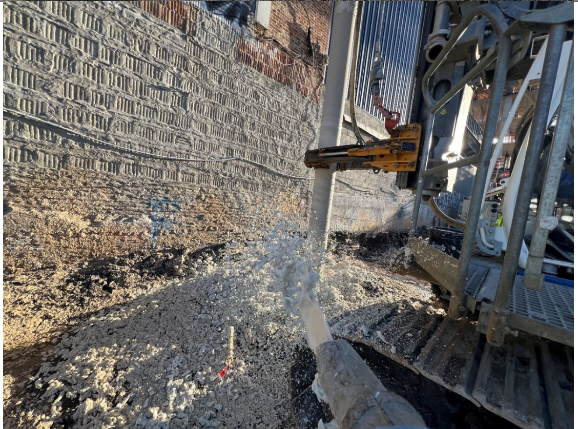
Photo 2- Representative photo of ATMOS foam applied during column installation.
