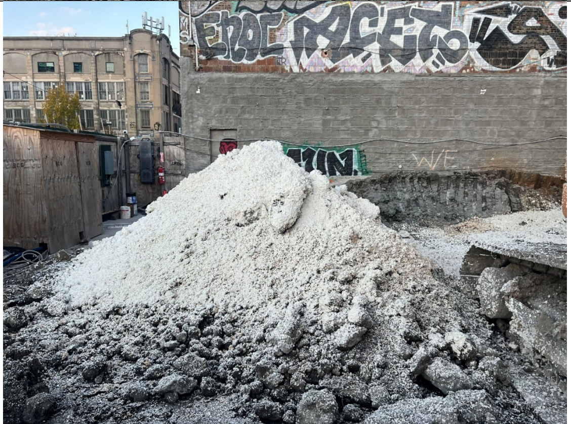
Photo 2- Representative photo of ATMOS foam applied to swell stockpile at the end of the day.
