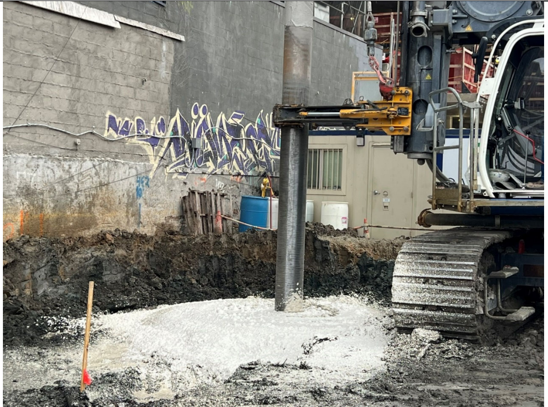
Photo 1- Representative photo of drilling an ISS column.
