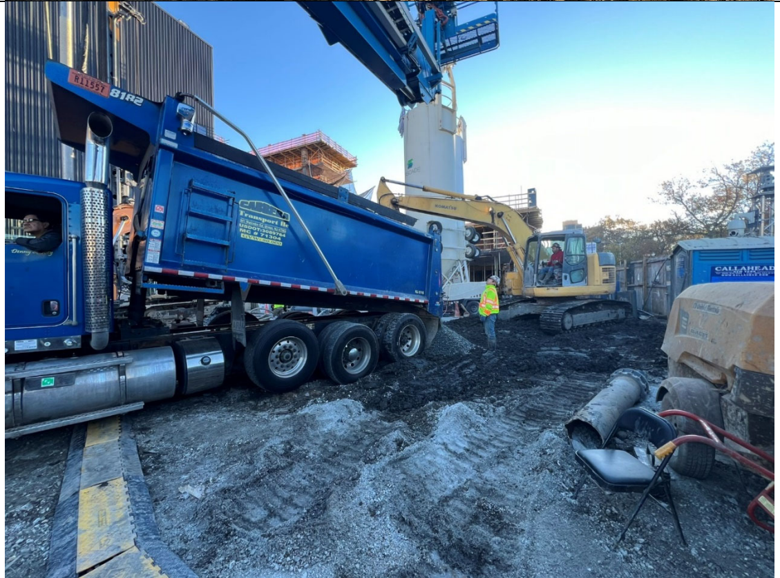
Photo 4- Representative photo of the stone delivery.
