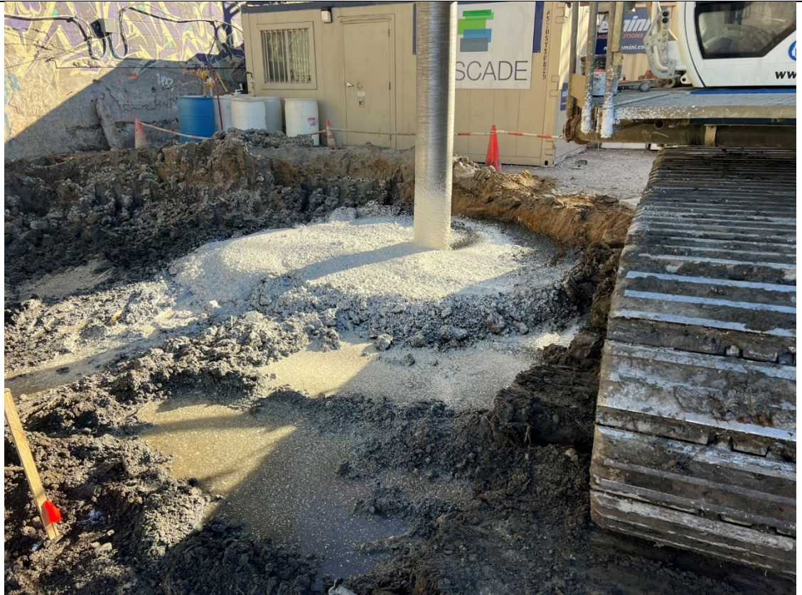
Photo 1- Representative photo of drilling an ISS column.
