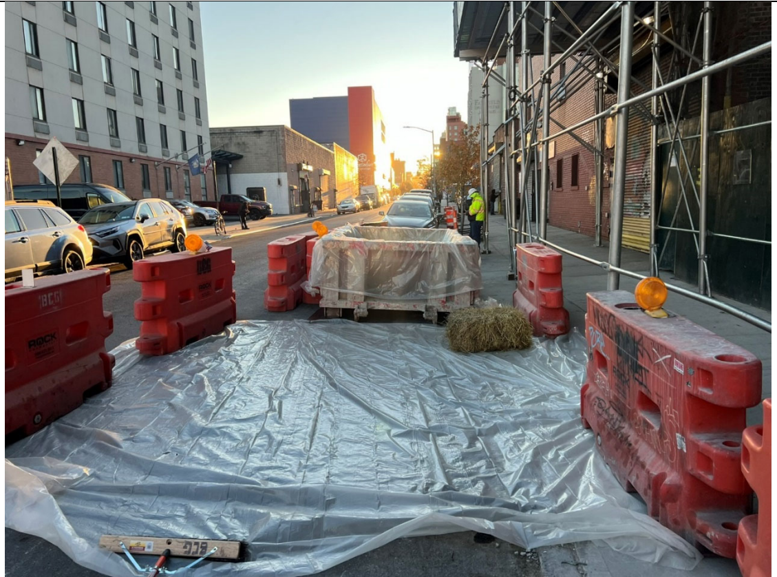
Photo 3- Representative photo of the concrete washout station.
