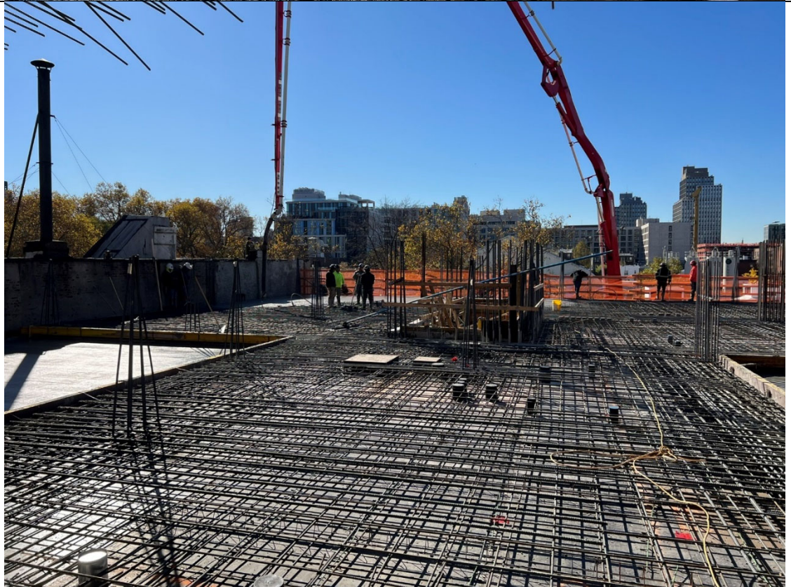
Photo 2- Representative photo of the concrete pour.
