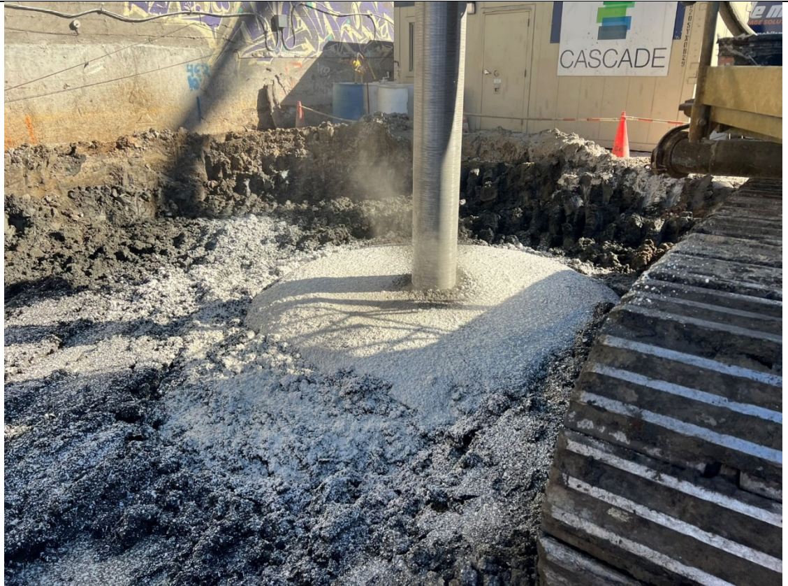
Photo 1- Representative photo of drilling an ISS column.
