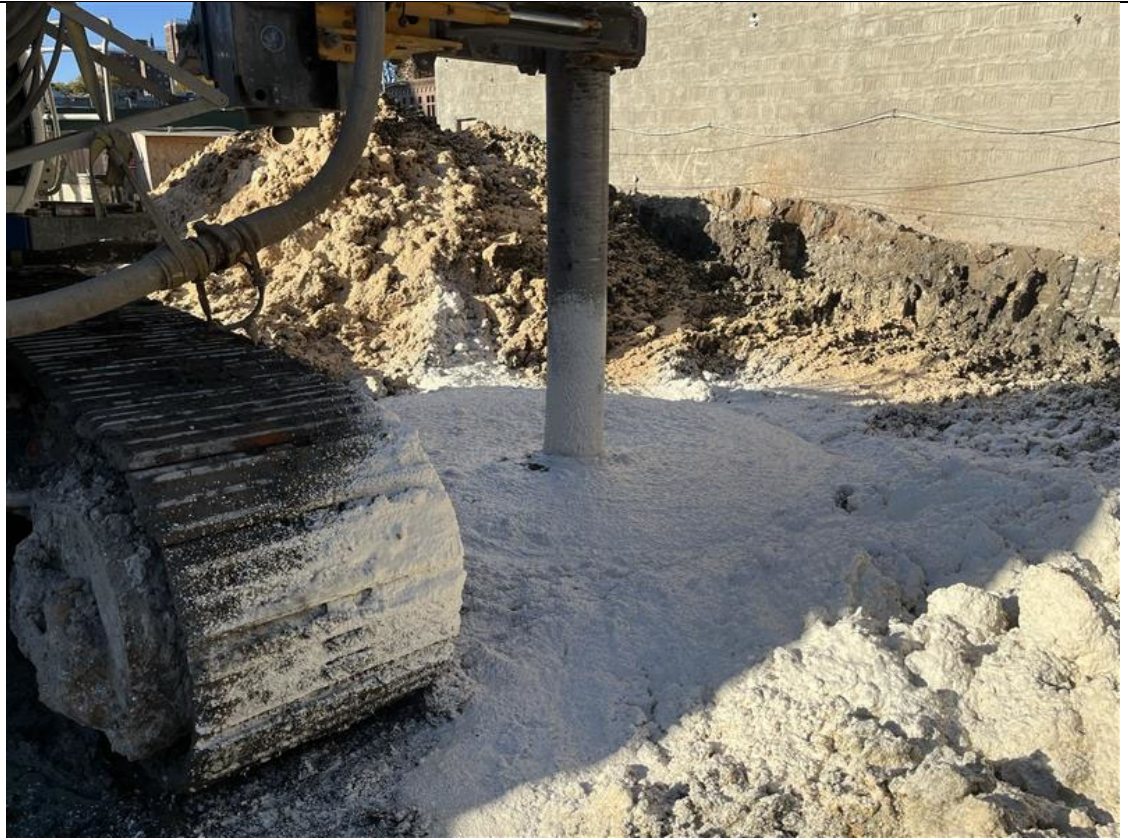
Photo 1- Representative photo of drilling an ISS column.
