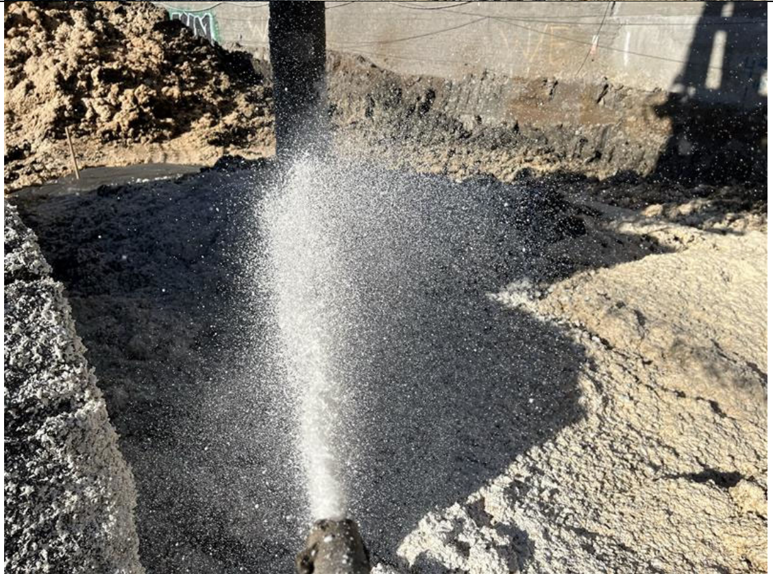
Photo 2- Representative photo of applying Atmos foam during ISS installation.
